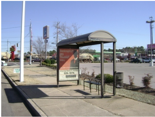
(a.) Bus shelter
