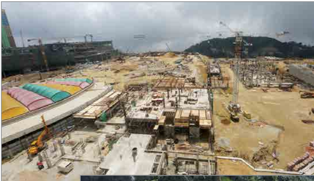
Construction progress at hill-top
