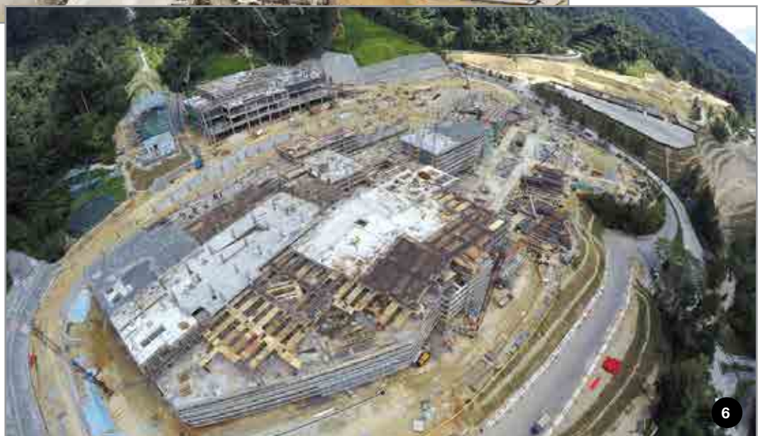
Construction progress at mid-hill
