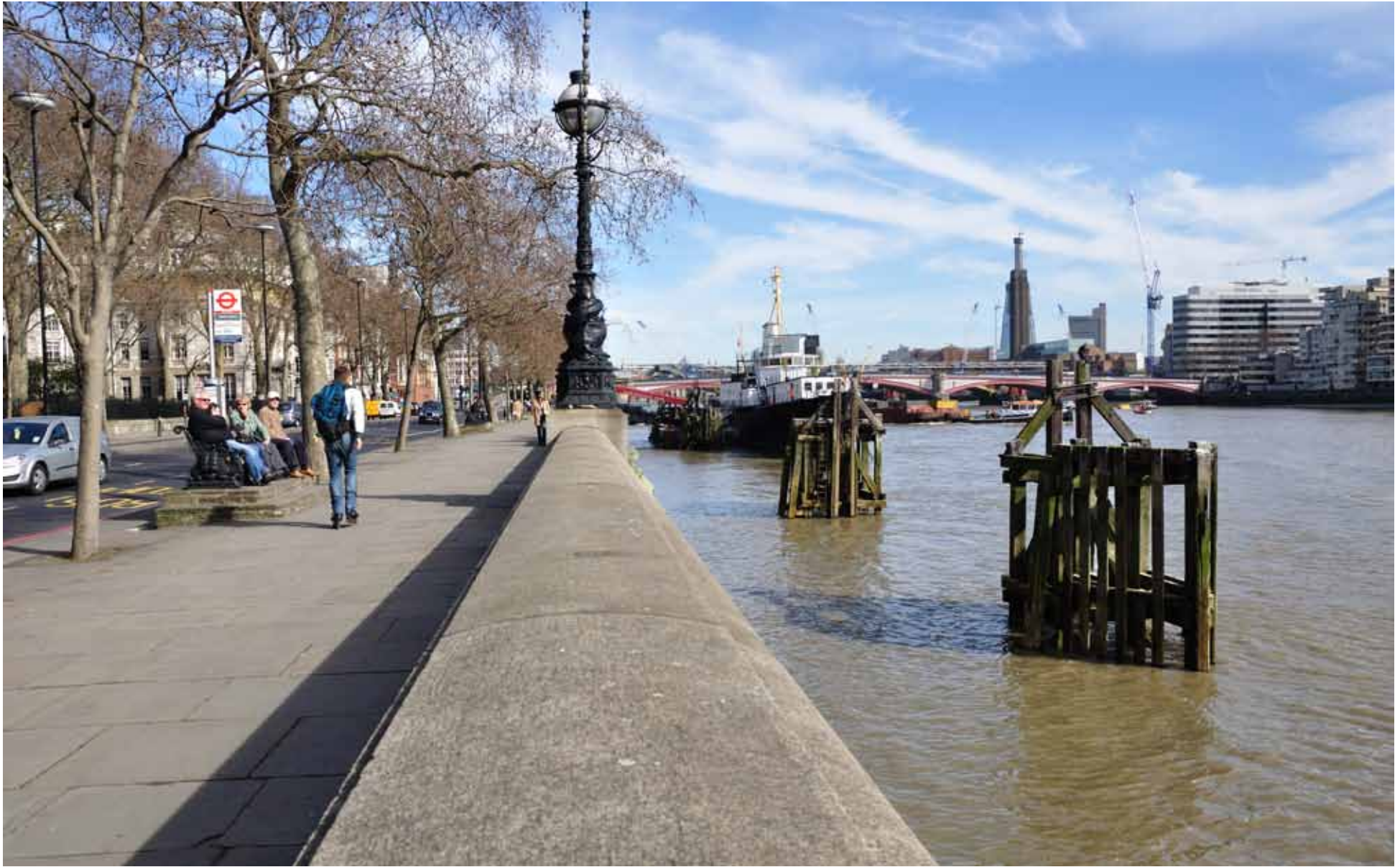
Blackfriars Bridge foreshore site
