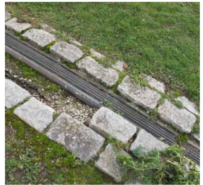
Mile End Bridge
