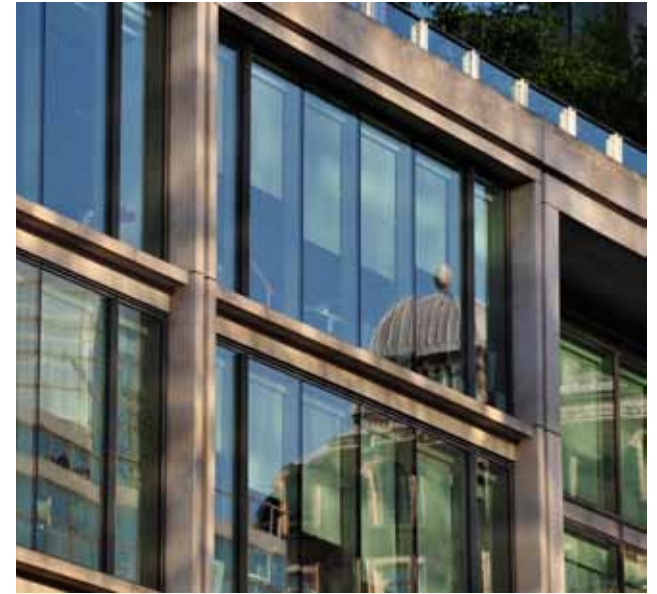
Buckingham Palace Road Roof Terrace
