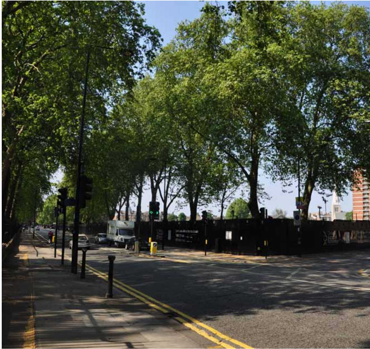
Chelsea Barracks site, Chelsea Bridge Road
