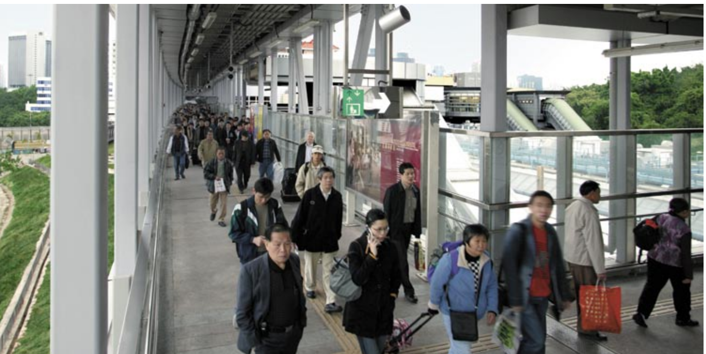
The Corporation continues to improve the station environment and arrangements for passenger flow at Lo Wu Station.
