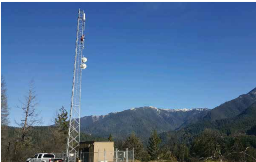
Joshua Hillman installing equipment on Áan Chúuphan Tower, Orleans, CA
