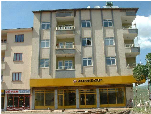
Fig. 8 The Dunlop building appears undamaged from the façade
