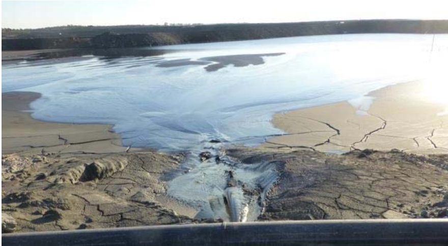
Fig. 3.8 Photo of thickened tailings disposal (photo courtesy of, A.Bjelkevick)
