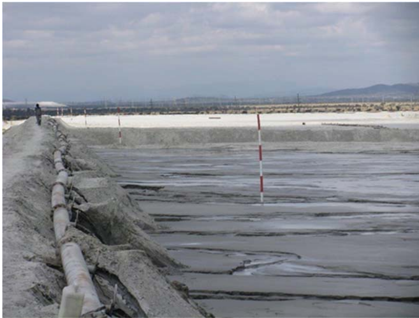
Fig. 3.1 Spigotting via apertures in the distribution pipe (McLeod and Bjelkevik 2017)
