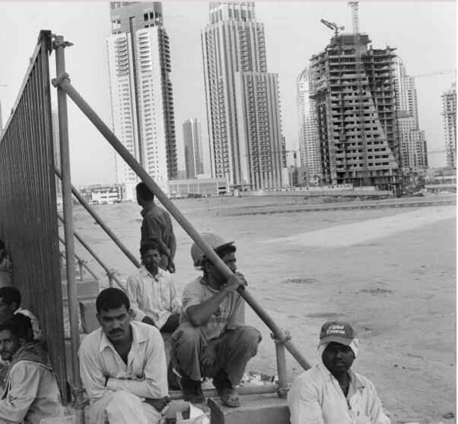
In front of the beach apartment complex they are helping to build, foreign workers wait for the bus that will take them home.
