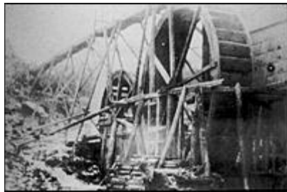
Mr. Scanlan (?) washing quartz for gold in front of a water-powered chusher at Brigus on August 13, 1886. (III/3.)
