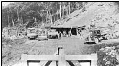
Indian Head mine, c. 1942. Ore slid down hill to loading platform and into waiting trucks (V/5.) Larger Version (27 kb)
