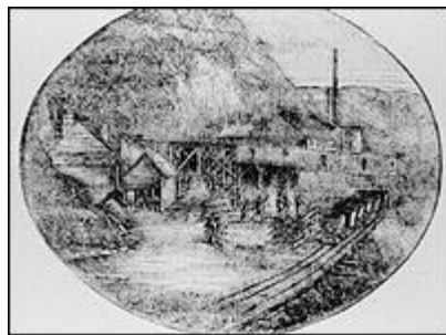
Engraving of Betts Cove c. 1878, printed on reverse side of Betts Cove Mining Company bills. Swansea cars and ore smelters are in foreground. (II/2.)
