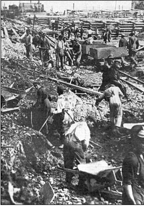
Opening up the Aguathuna limestone quarry, c. 1912. Beginnings of pier construction can be seen in the distance. (V/7.)
