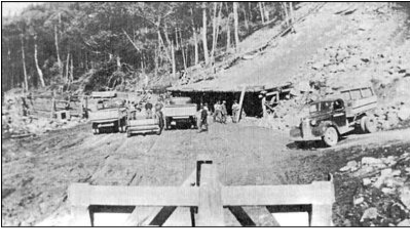
Indian Head mine, c. 1942. Ore slid down hill to loading platform and into waiting trucks (V/5.)
