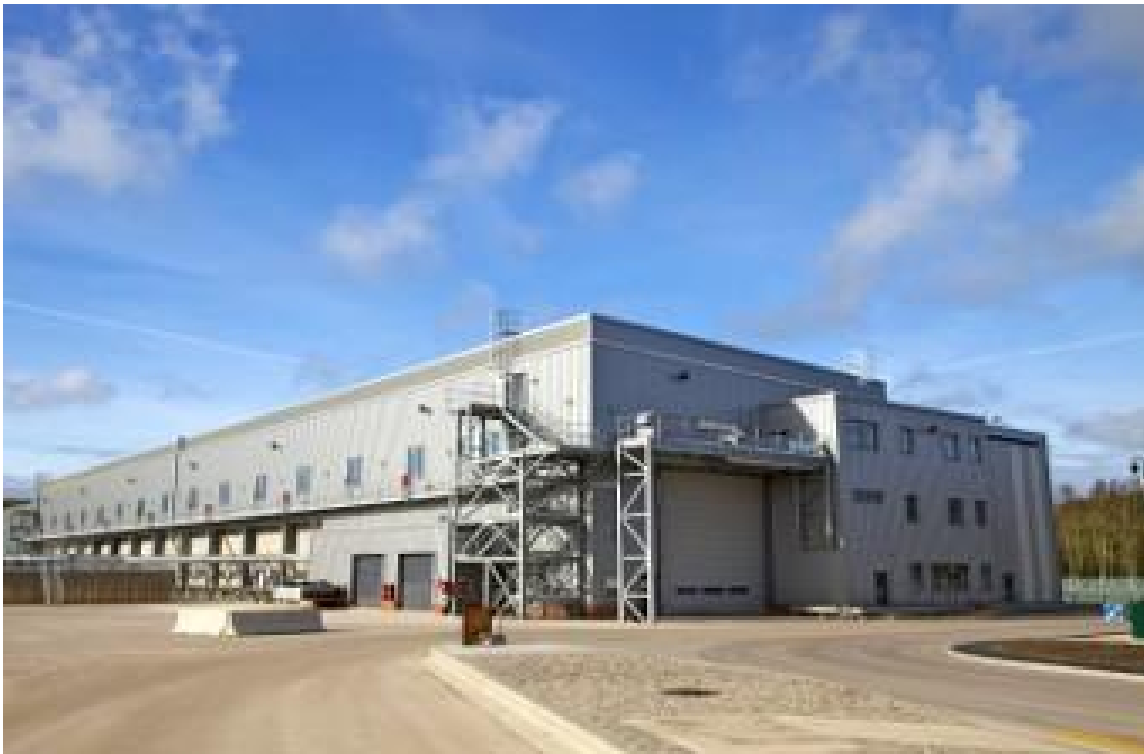
Figure 24 shows an external view of the Shanks MBT facility at Hespian Woods, Cumbria. This facility has a design throughput of around 75ktpa 66 .
