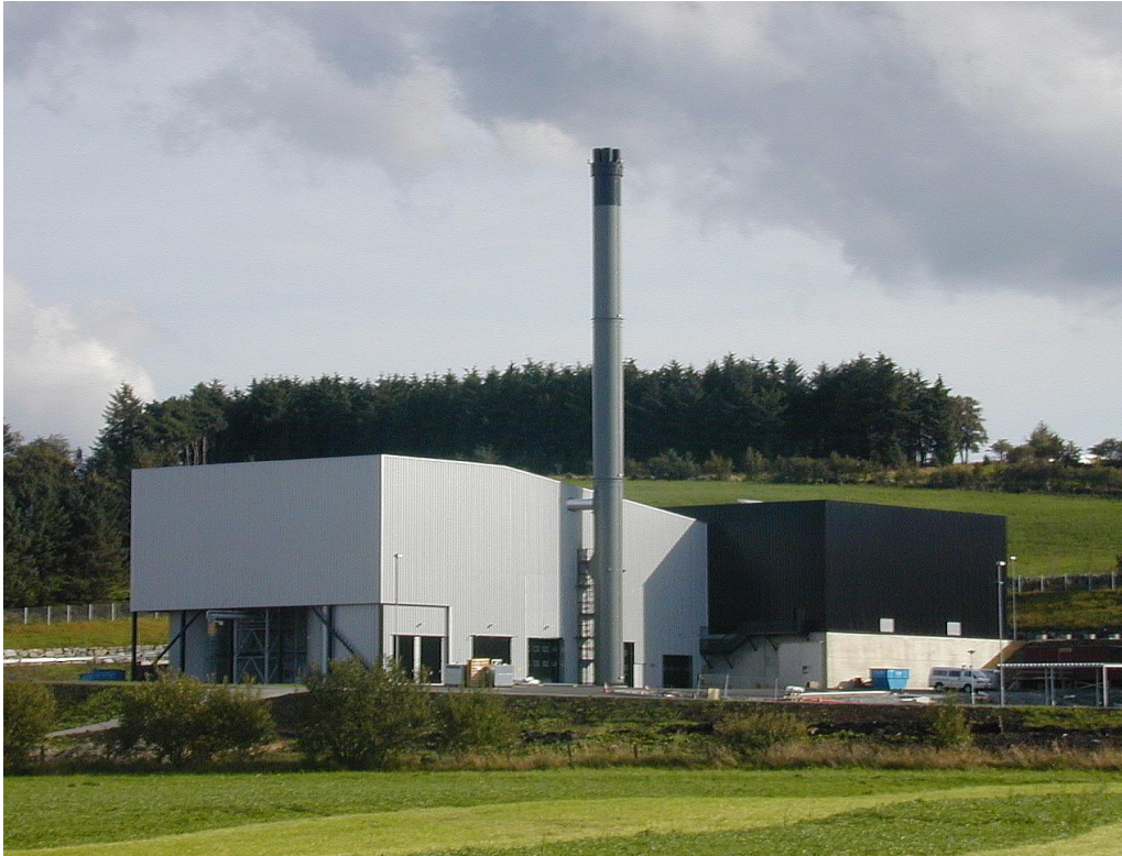
Figure 3 – A typical two-stage gasification facility
