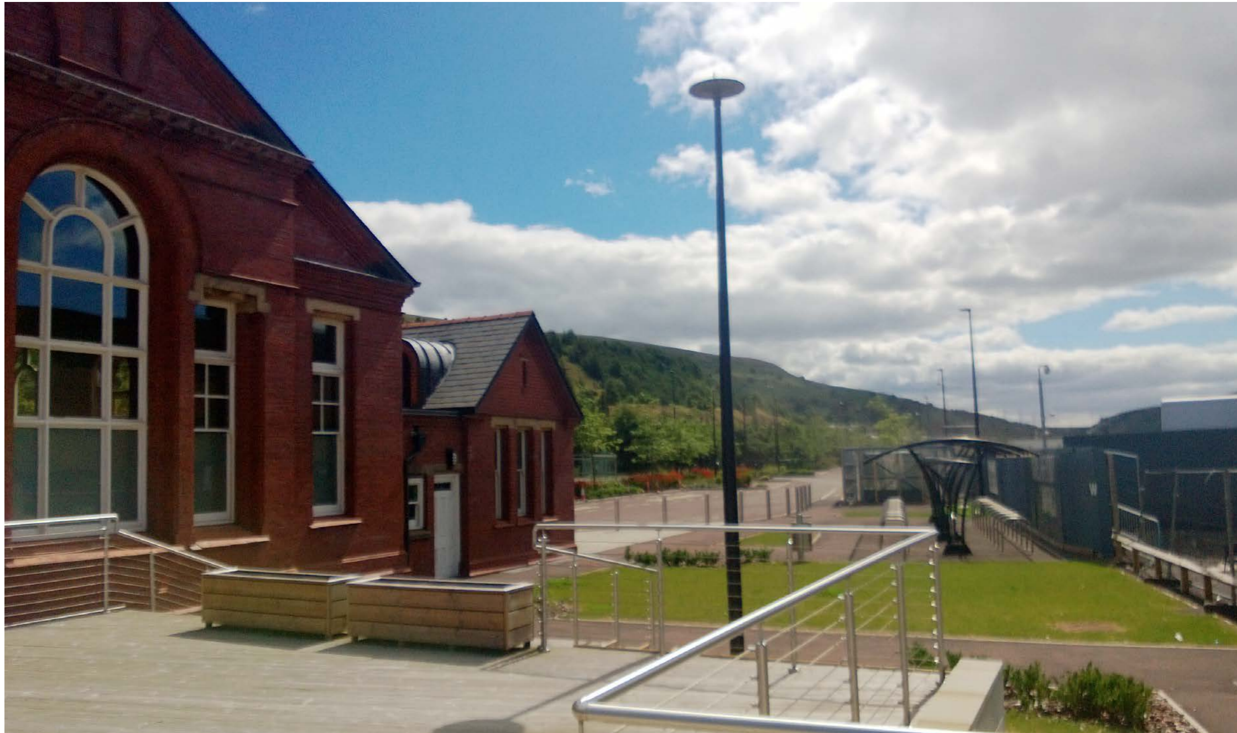
View south towards Network Rail land from Gwent Archive. Highlights the relationship between car parking, cycle parking and architectural context.
