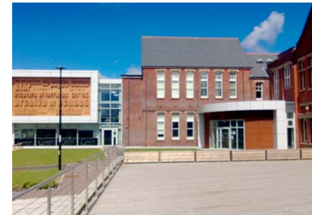
View north from close to the proposed railway station which shows the high quality refurbishment and new public space in front of the Gwent Archive. The proposed railway station will need to take account of this in terms of use of materials and pedestrian movement.
