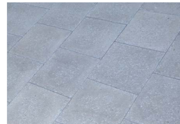
Precast concrete paving
