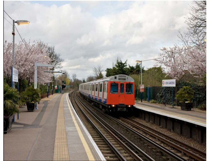
High quality landscaping and planting at Kew Gardens station creates a sense of arrival that reflects its location.
