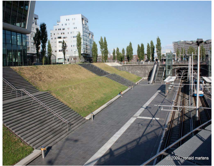
The new Reitlandpark railway station in a new district of Amsterdam demonstrates how a station separated by a change of level can be integrated into its surrounding urban context.
