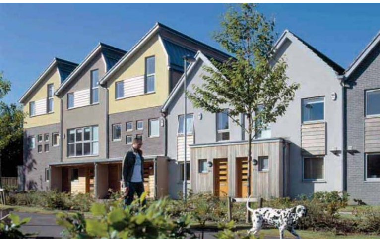
Upton is characterised by the density of units and public realm design that promotes walking and cycling over the private car.
