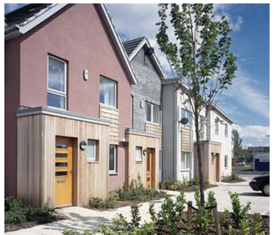
Larger family housing is designed to fit into a high density layout and overlooks public open space.
