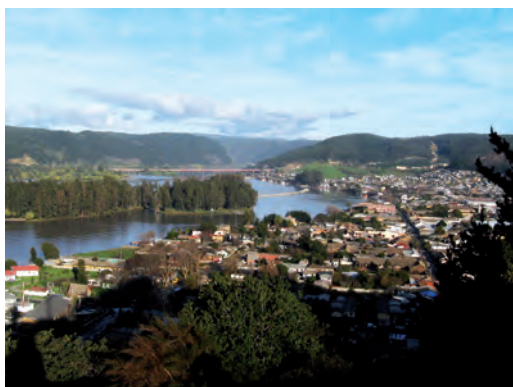
Figure 5.5 A and B, Before and after. Overview of the damages caused by tsunami in Constitución
