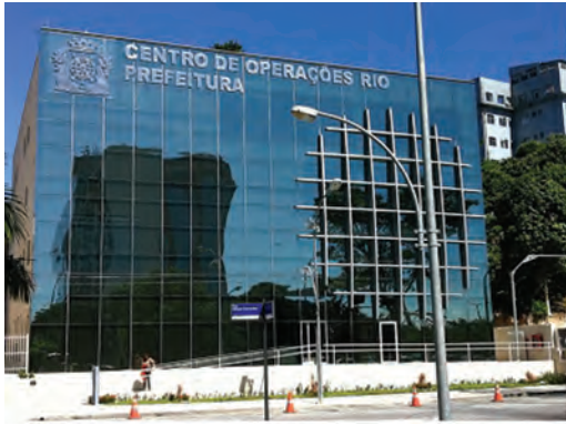
Photo 4.11: CO-RIO, City Government Operations Center
