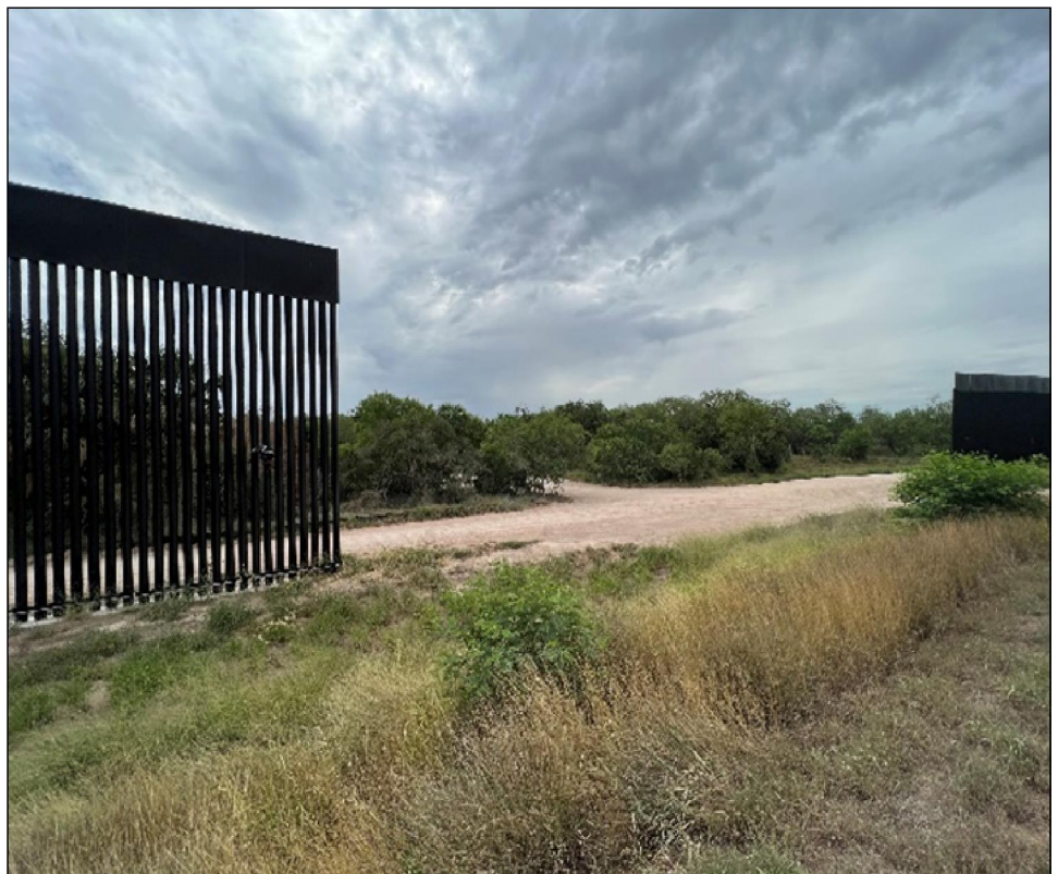
Figure 12: Opening Between Installed Panels in Texas (July 2022)
