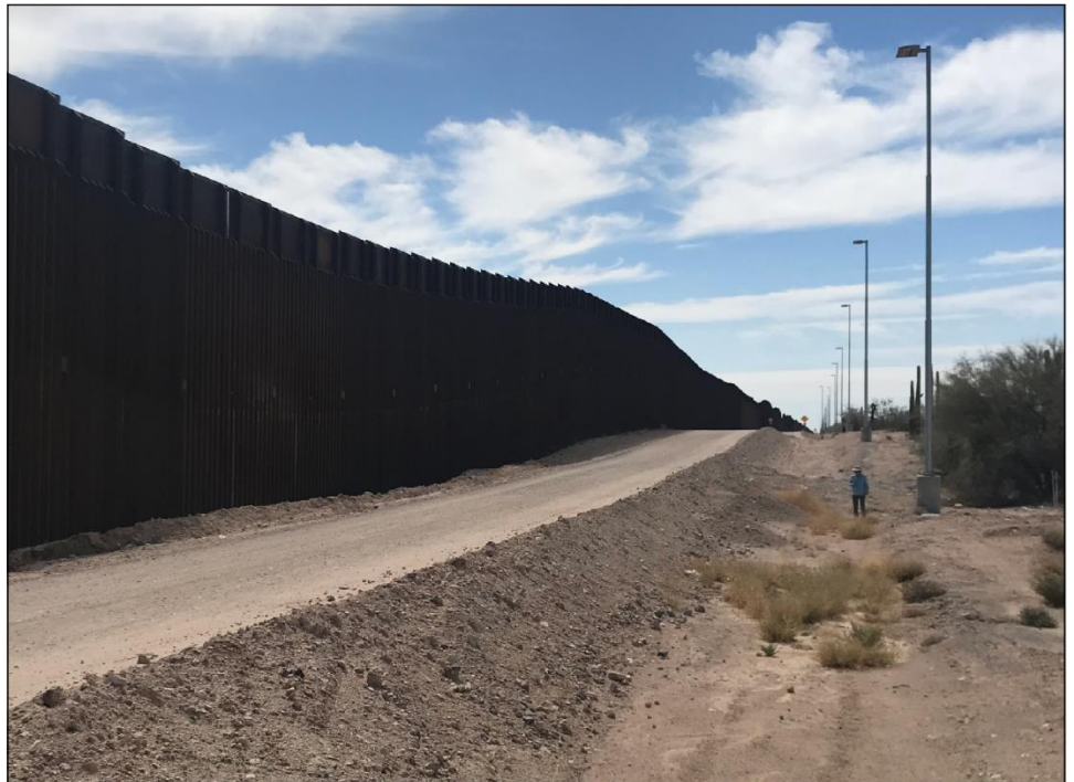
Figure 7: Raised Patrol Road above the Desert Floor in Arizona (May 2022)
