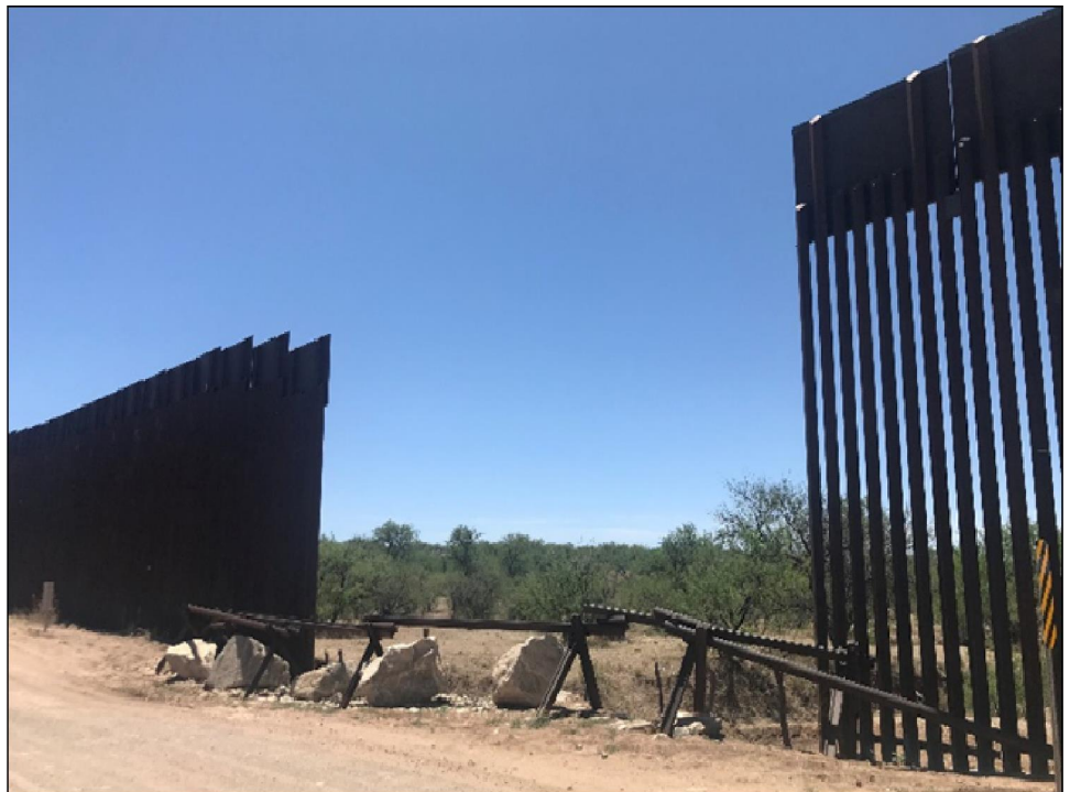
Figure 6: Incomplete Border Barrier in Arizona, with Opening (May 2022)
