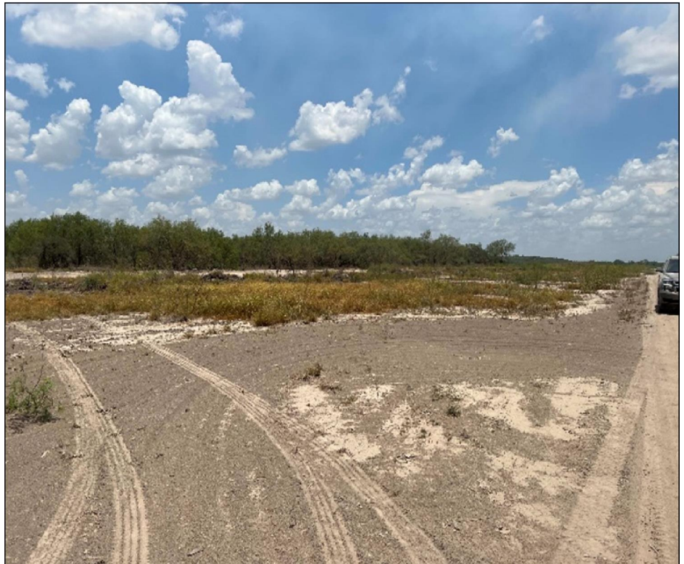
Figure 10: Barrier Project Site Cleared of Native Vegetation in Texas (July 2022)
