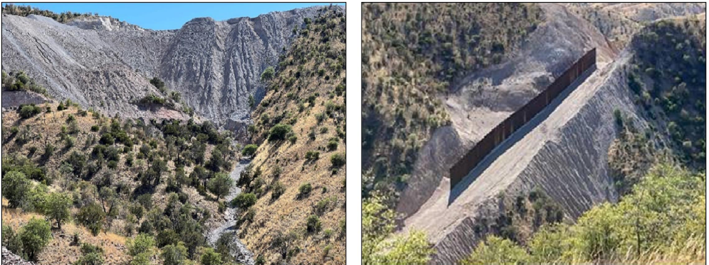
Figure 11: Erosion on the Coronado National Forest in Arizona (May 2022)
