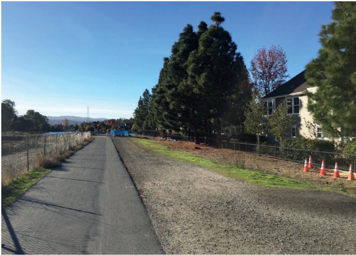
Photo 1 - View of project site from Levee Pedway, looking west
