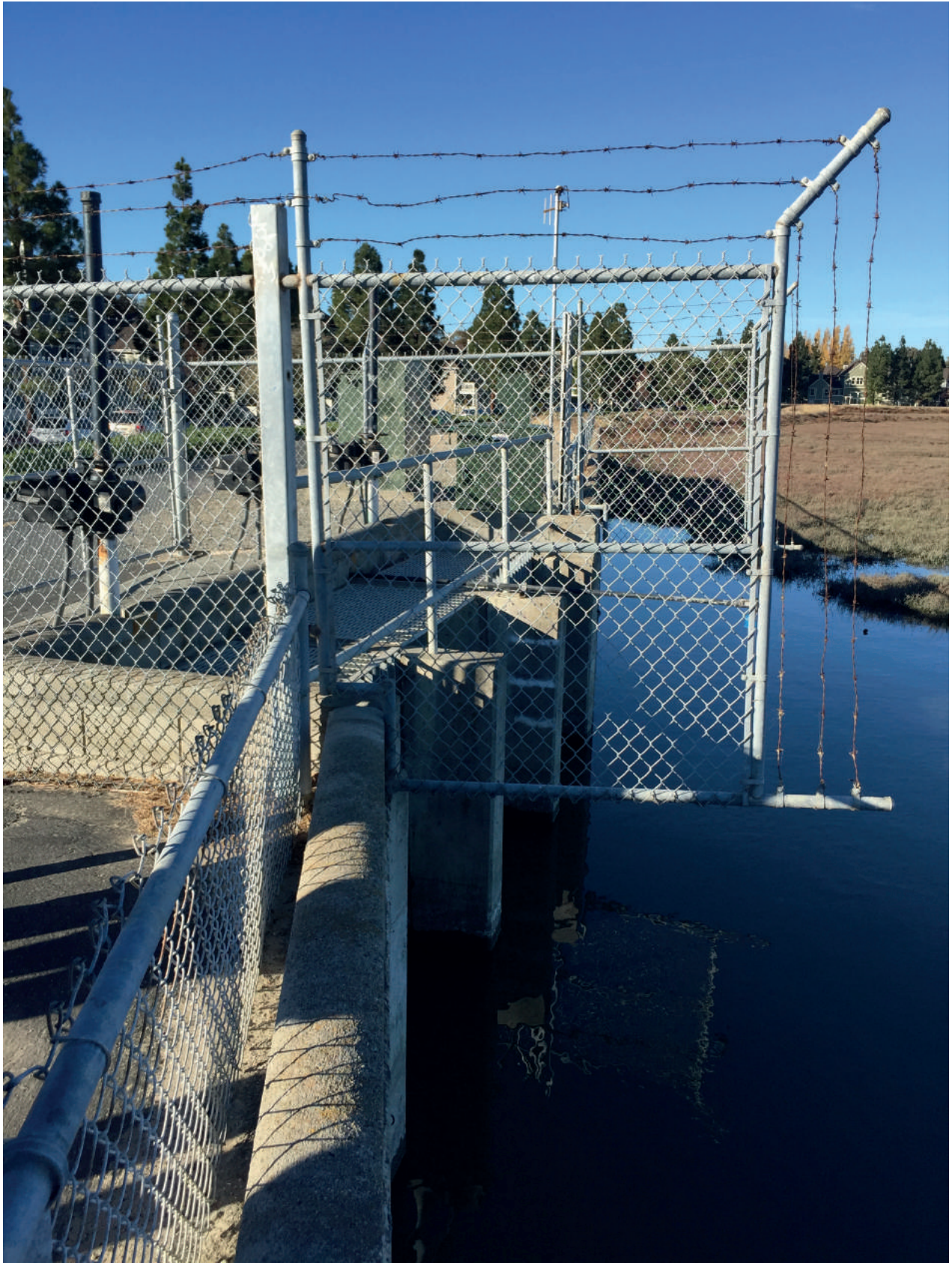
Photo 3 - View of western intake structure from Levee Pedway, looking north
