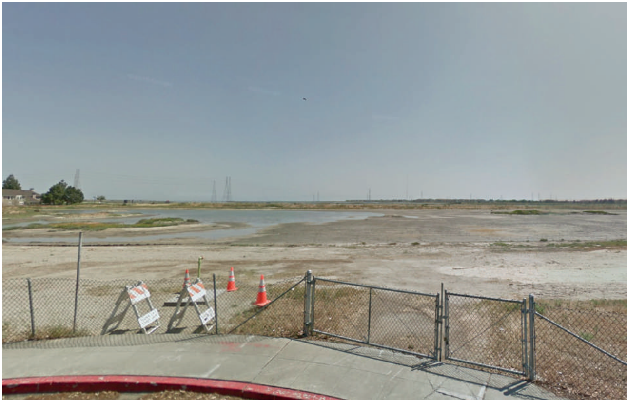
Photo 7 - View of Sea Cloud Phase II site from Sea Cloud Park (Sea Cloud Drive), looking east
