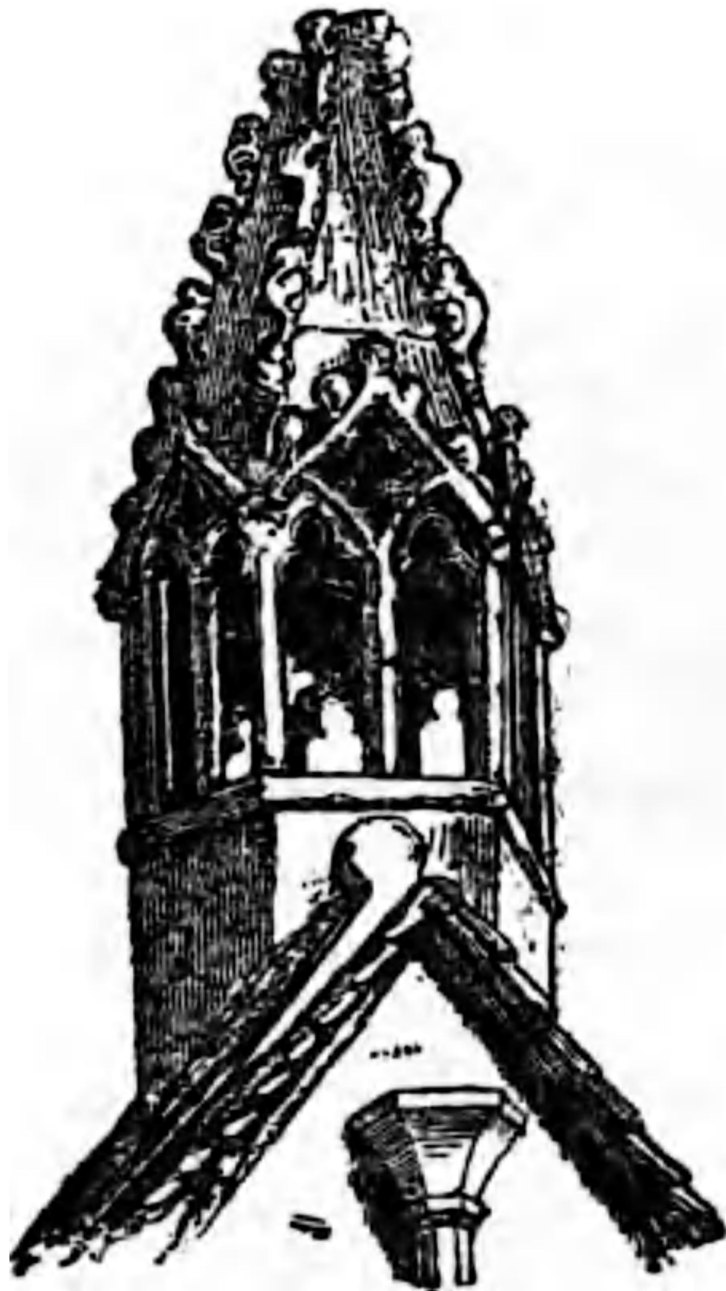
OLD CHIMNEY FORMERLY ON THE SOUTH SIDE OF WITNEY STREET.
