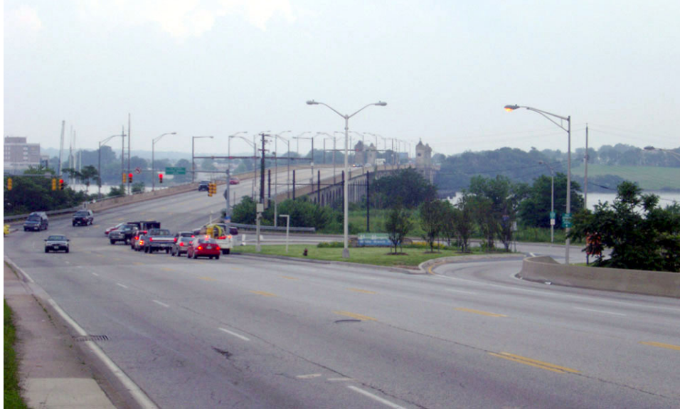
Figure 78. Example of a jughandle intersection.
