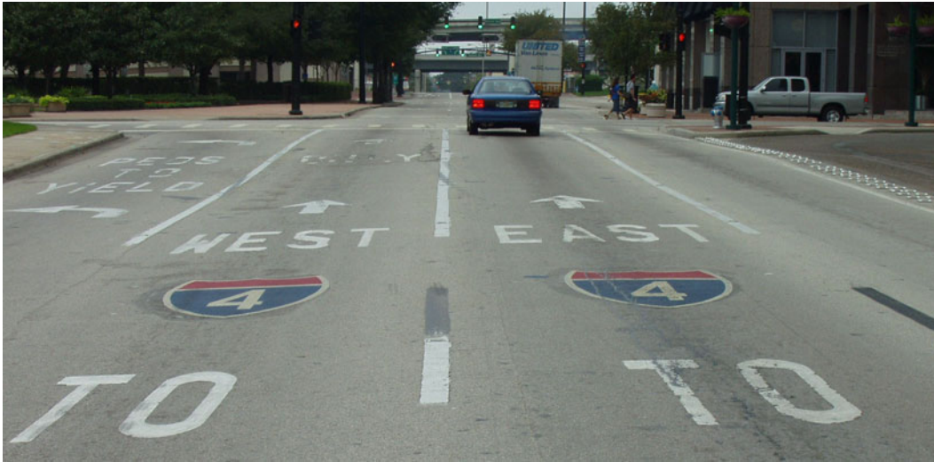
Figure 42. Example of pavement legends indicating destination route numbers (“horizontal signage”)
