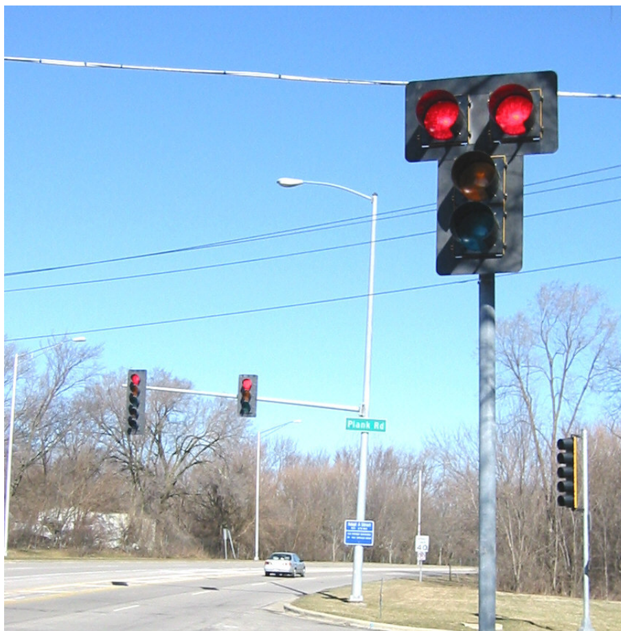
Figure 113. Signal head with a double red signal indication.
