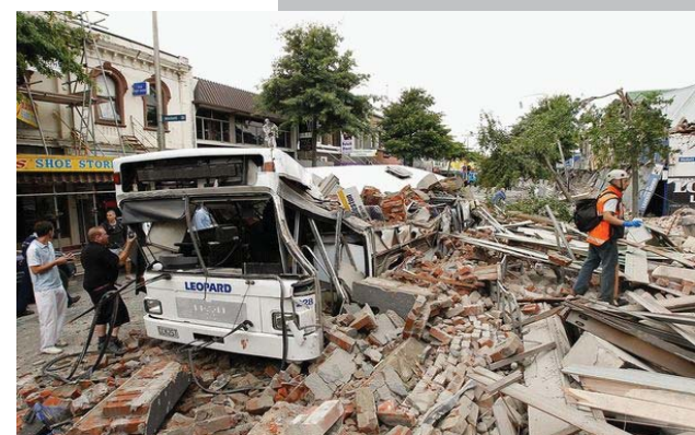
Christchurch, NZ, September, 2010 – Citizens and responders survey the aftermath of the magnitude 7.1 earthquake that struck 30km west of Christchurch, NZ. Most structural damage was due to unreinforced masonry (URM) as shown. - GettyImages
