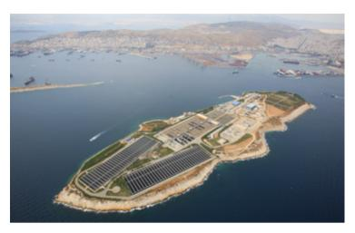
The Psyttalia WWTP is the main wastewater treatment plant in the greater Athens area, receiving an average wastewater flow of approximately 730,000 m<sup>3</sup>/d. The Psyttalia WWTP capacity is 5.600.000 p.e., being one of the biggest WWTPs in Europe and worldwide.
