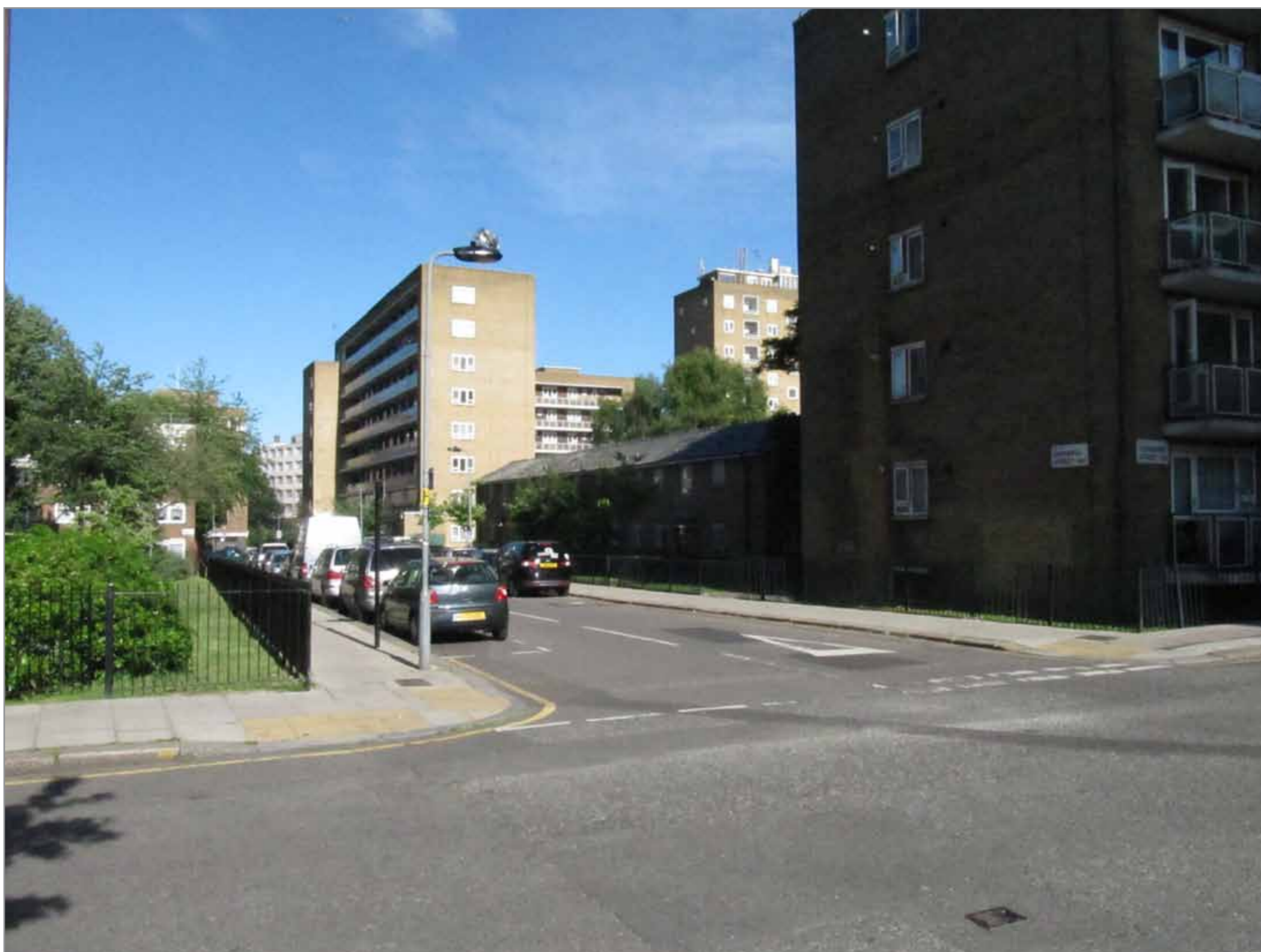
View of the existing Staveley block from Varnell Street
