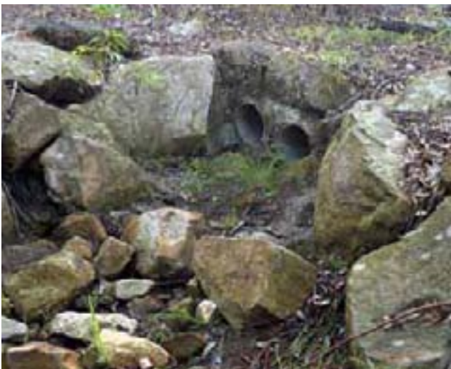
Figure 18: Sandstone armouring of the creek preventing erosion and reducing the force of the water
