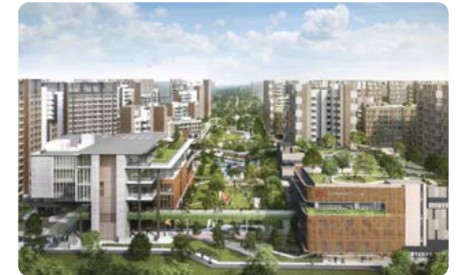
Image of fully constructed Tengah Town, a smart city in Singapore
