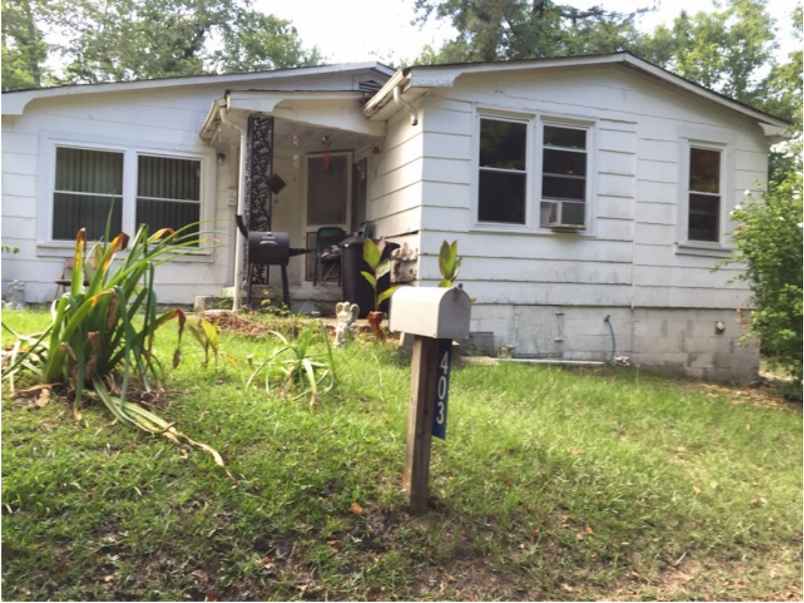
SCOPE home in St. Matthews, SC July 2016
