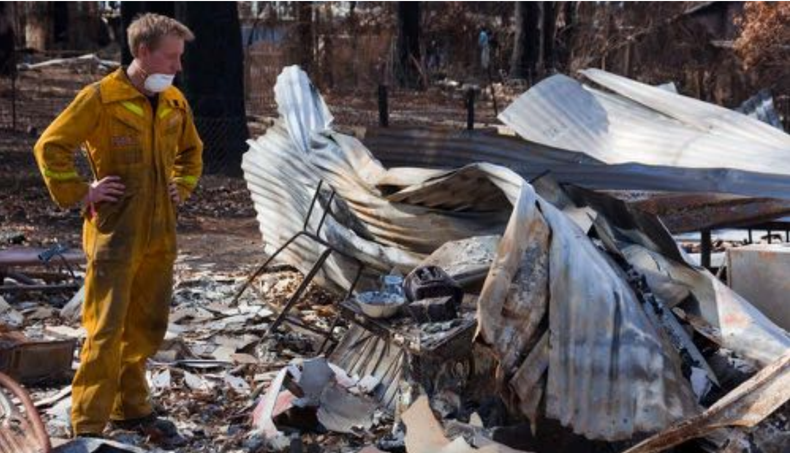
Figure 12: A firefighter observes the wreckage of a home in Kinglake, Victoria.
