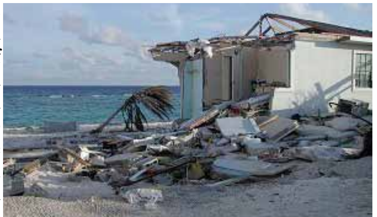
Damage from Hurricane Ivan
