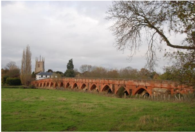
Views towards Barford Bridge and the church at Great Barford from Barford Road, close to the border with Bedford Borough
