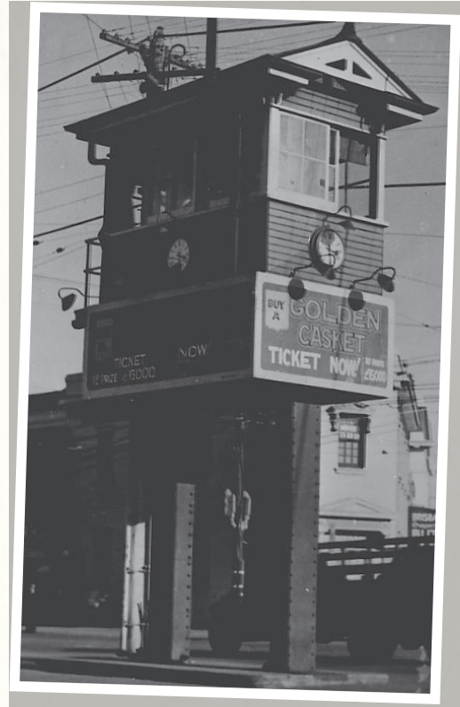
Tram Control Room, Woolloongabba Fiveways, 1930s, Brisbane City Council, Negative Number BCC-B120-30757
