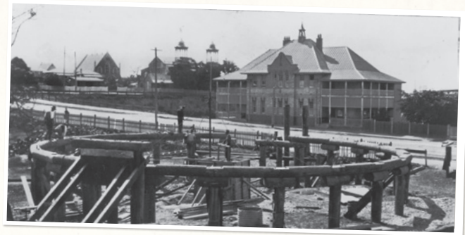
Construction of a railway turntable in Main Street, Woolloongabba, 1921, State Library of Queensland, Negative Number 37394
