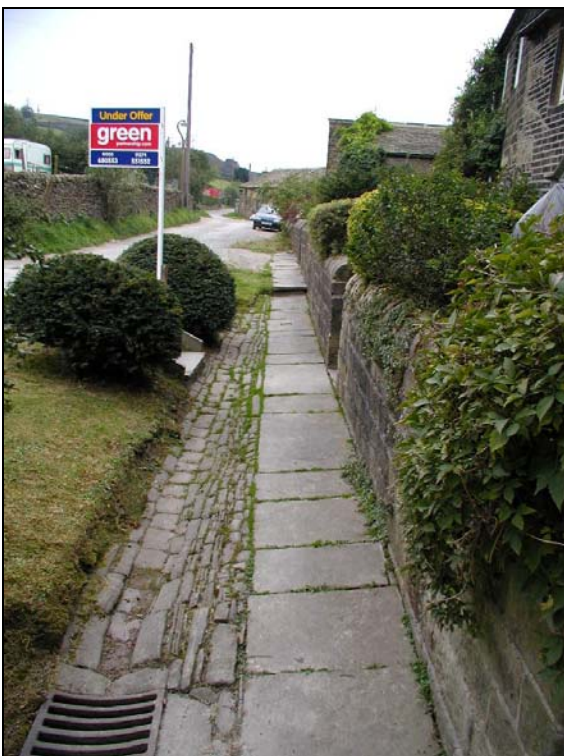
Above: Hill Top Road is unmade and is in a poor condition in places, though its country lane character is important to the feel of the conservation area. Left: Flagged pavement and setted gutter in front of 20-21 Hainworth. Below: composite view of Hill Top Road from the Green. Boundary walls define the funnel shape of the roadways and the buildings are set at irregular angles. Note the ending of the tarmac and the surfacing of Hill Top Road with a grey gravel which does little to complement the stone of the buildings, pavement and walls.
