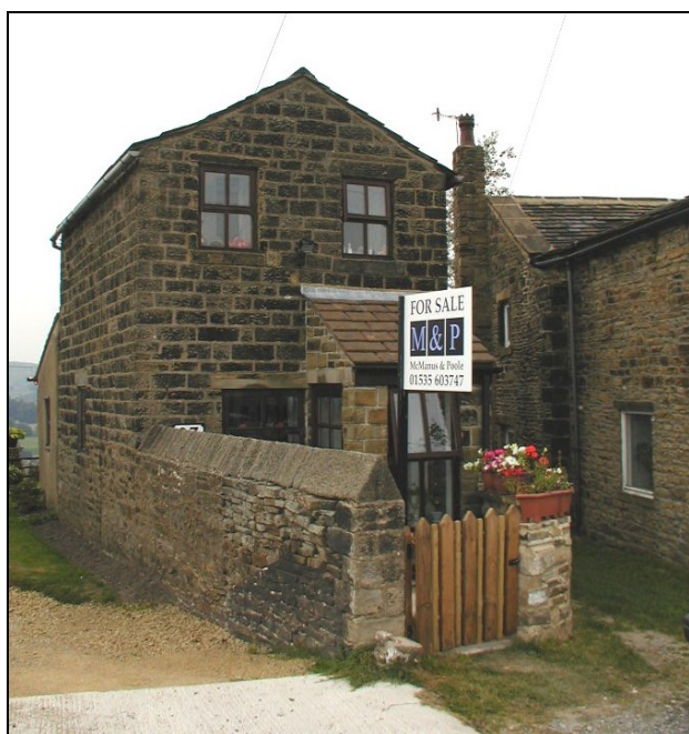
23 Hainworth (key unlisted building) is thought to have been built for the Hainworth Co-operative Society in the 1850s.
