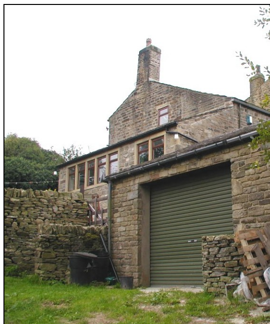
This gable-end extension matches the older building in terms of materials and plain stone mullioned window margins. Like the garage in the foreground, which also uses local stone, it is sensitively sited away from the main elevation of the building.
