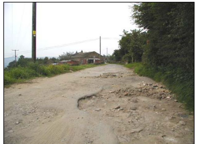
Above: Hill Top Road is unmade and is in a poor condition in places, though its country lane character is important to the feel of the conservation area. Left: Flagged pavement and setted gutter in front of 20-21 Hainworth. Below: composite view of Hill Top Road from the Green. Boundary walls define the funnel shape of the roadways and the buildings are set at irregular angles. Note the ending of the tarmac and the surfacing of Hill Top Road with a grey gravel which does little to complement the stone of the buildings, pavement and walls.
