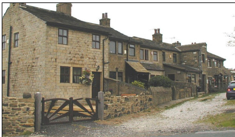
The varying boundary treatments at 32-38 Hainworth (and lack of them) reflect the organic growth of the row and the squeezing in of the buildings between a fields boundary and the right of way. The modern walls to the left are out of keeping.
