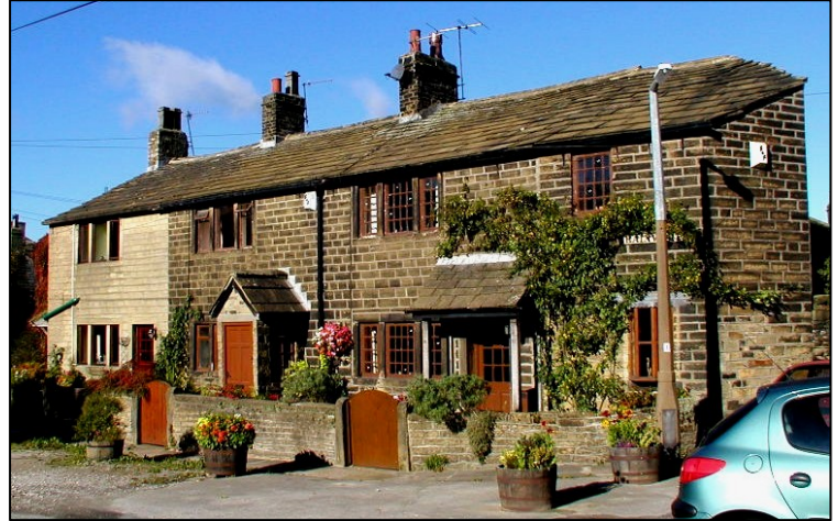
12-15 Hainworth is Grade II Listed as a good early example of a row of cottages. The row is prominently placed and is of considerable townscape value.
