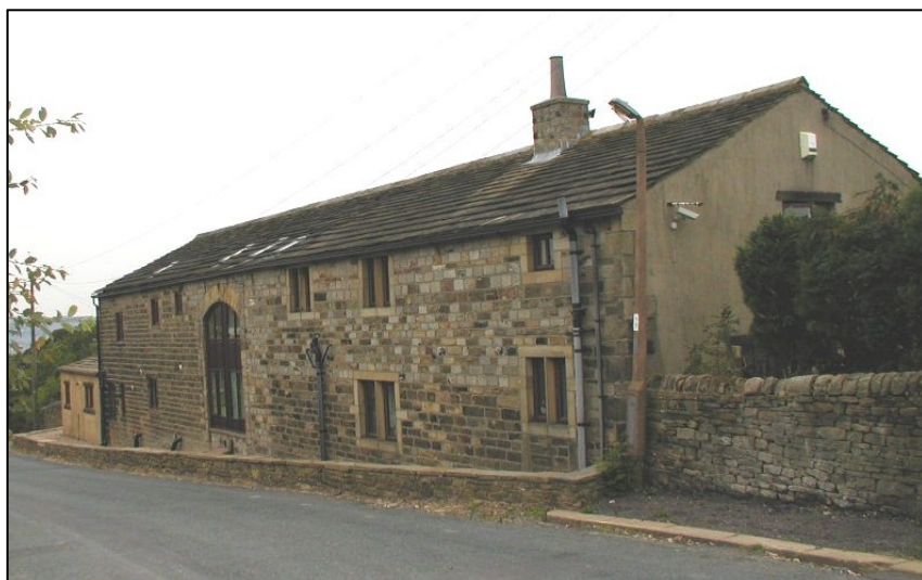
Hainworth Farm Cottages (unlisted), a former barn which has lost much of its original character through unsympathetic conversion. Fortunately the roadside elevation is the least altered.
