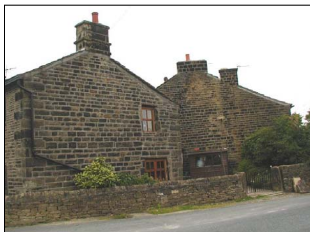
Stone boundary walls make an important contribution to the street scene and harmonise well with the stone of the buildings.
