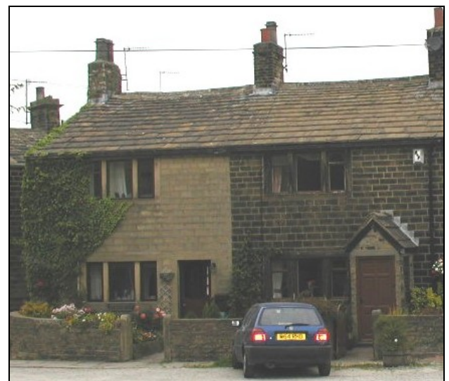
Stone cleaning can create unwanted demarcations between buildings and undermine their coherence.
