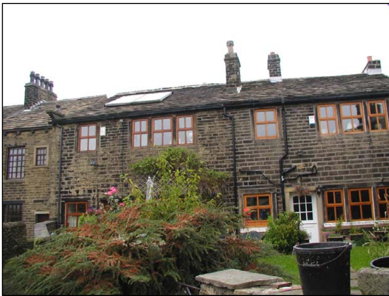
10-11 Hainworth were probably weavers' cottages/workshops as the fenestration maximises the southern prospect of this elevation.
