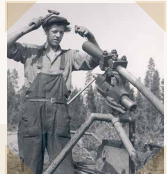
The ropeway conveyor between the Kristineberg mine and Boliden was built in 1943.
