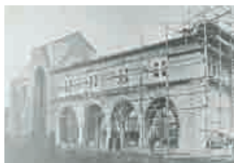
Building of Christ Church Bexley Heath, 1873
