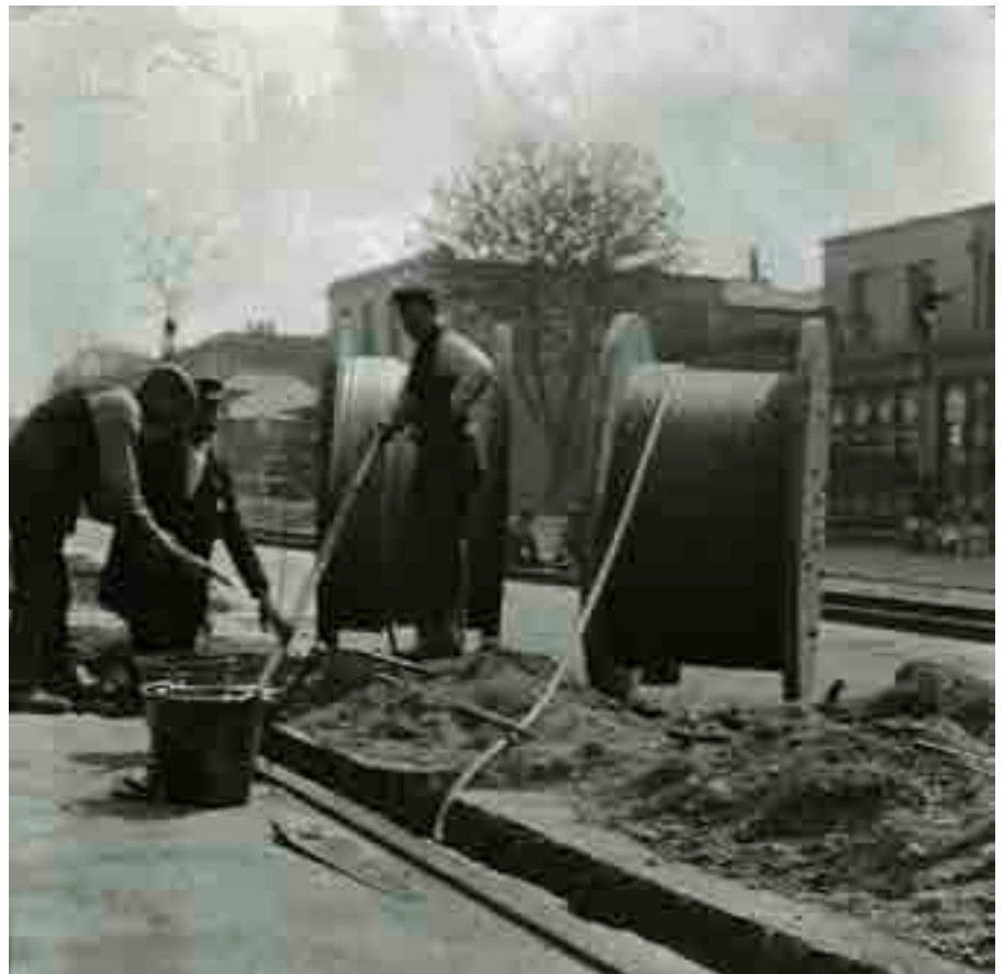
Workmen laying electricity cable in the Broadway Bexleyheath, early 20th Century
