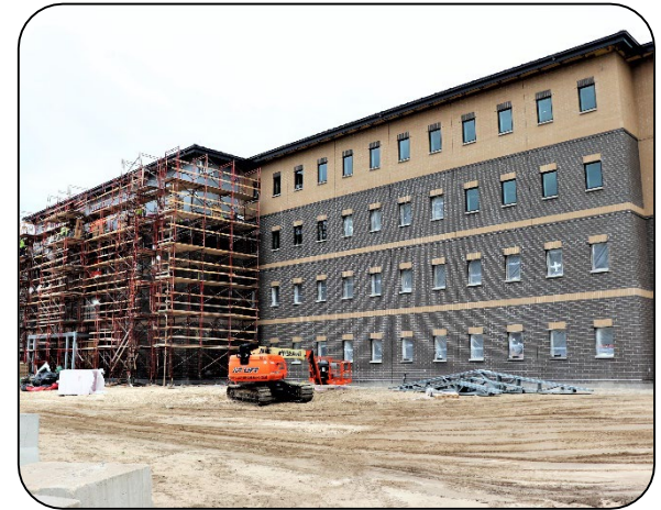
Fort McCoy Transient Training Barracks construction project
