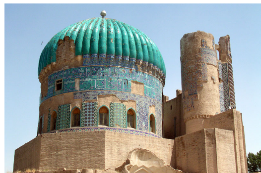
Figure 13: Balkh, the Khwadja Parsa Mausoleum, baked brick and earthenware from the Timurid monument, end of 15th century A.D. The building is seen from ¾ back showing one of the round tower of the "iwān" and the ribbed dome covered with blue earthenware surmounted by two drums, of which the lowest has windows.
