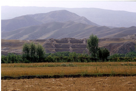
Figure 52: Surkh Kotal, the site and its terraces seen from the cultivated fields, east to west.
