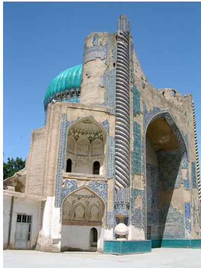
Figure 14: Balkh, the Khwaja Parsa Mausoleum, construction from the Timurid period, end of 15th century A.D., made of baked brick and covered with earthenware.
