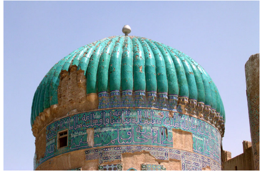
Figure 15: Balkh, the Khwaja Parsa Mausoleum, detail of the ribbed dome showing the damaged or destroyed areas after the 1970s restoration.
