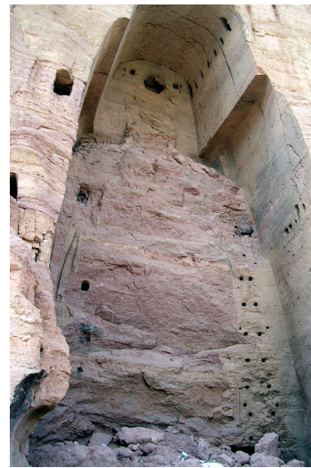
Figure 27: Bamiyân, the niche of the great 55 m Buddha statue. Photograph after the explosion by the Taliban. The cavities under the forearms show the built of a statue essentially carved into the rock.
