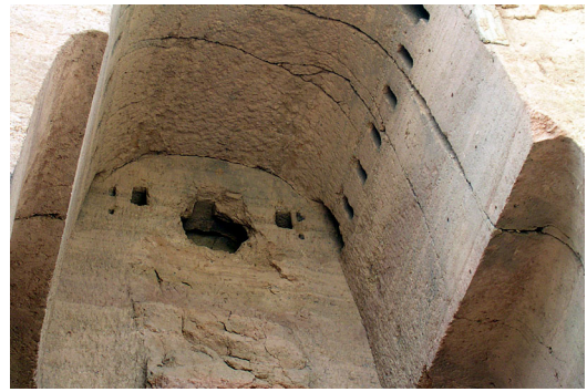
Figure 30: Bamiyân, the niche of the 55m Buddha statue. The high part of the trilobe niche with details of the central lobe, which consisted of a large cavity in the back part of the wall (North); that used to serve as the door giving access to the Buddha statue's head. The rows of holes seen on the lateral sides served as anchors for beams holding balconies.
