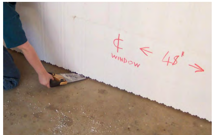
Figure 19 – Trimming the first course of block with a hand saw
