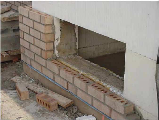
Figure 24 – Laying standard brick veneer on the brick ledge support
