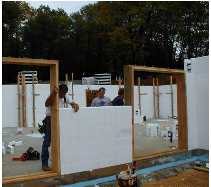
Figure 5 – Install window and door bucks
