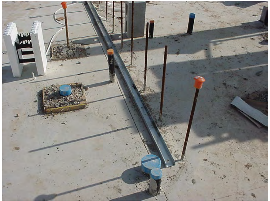
Figure 4 – Securing a metal track to a concrete slab
