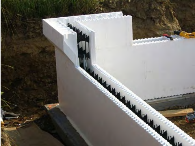
Figure 22 – Amvic brick ledge form installed as a single course
