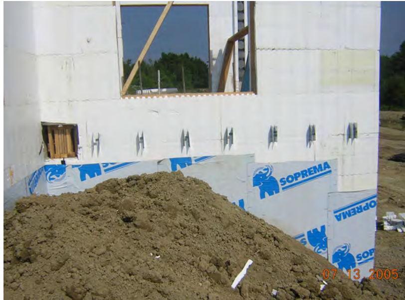
Figure 4 – Self-adhered waterproofing membrane installed and ready to be backfilled
