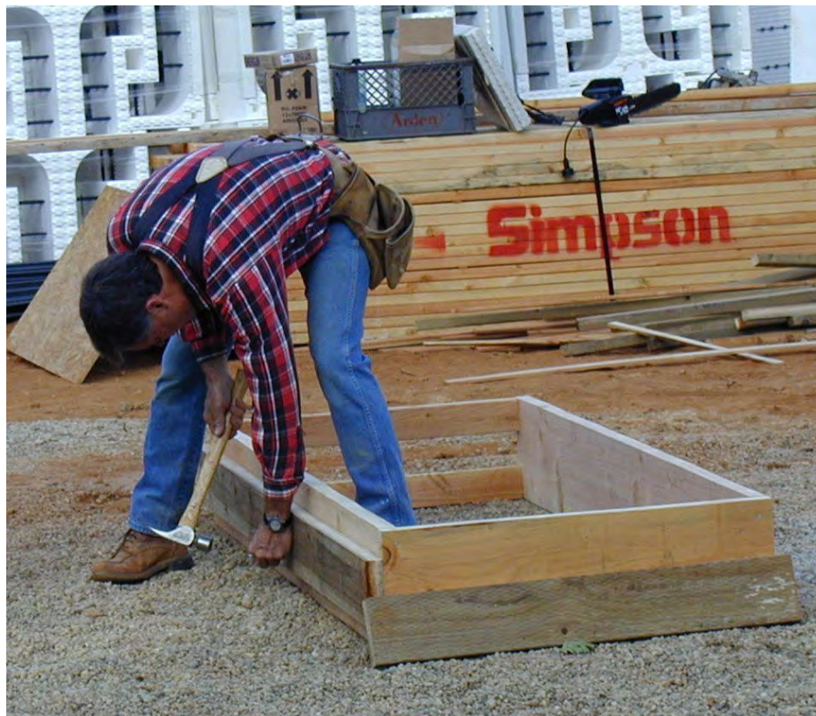
Figure 1 – Constructing your window/door bucks
