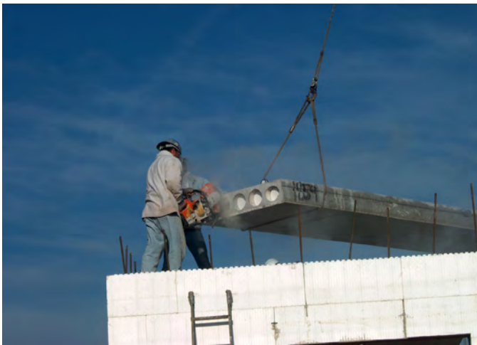
Figure 35 – Maneuvering a precast hollow core slab for placement on an ICF wall
