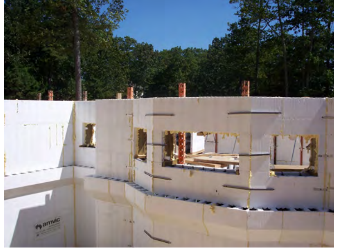
Figure 23 – Completed brick ledge installation for exterior brick veneer support
