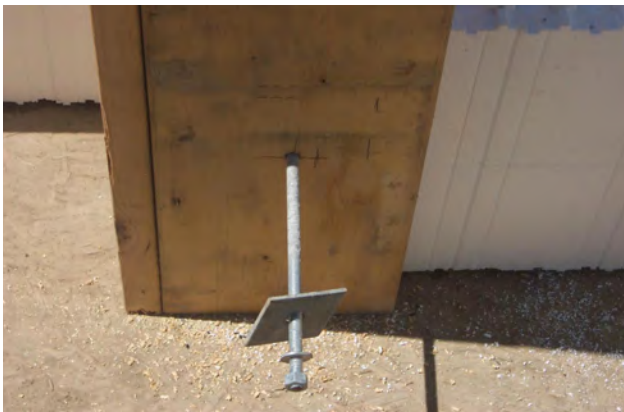
Figure 8 – Inserting the threaded rod through the drilled holes
