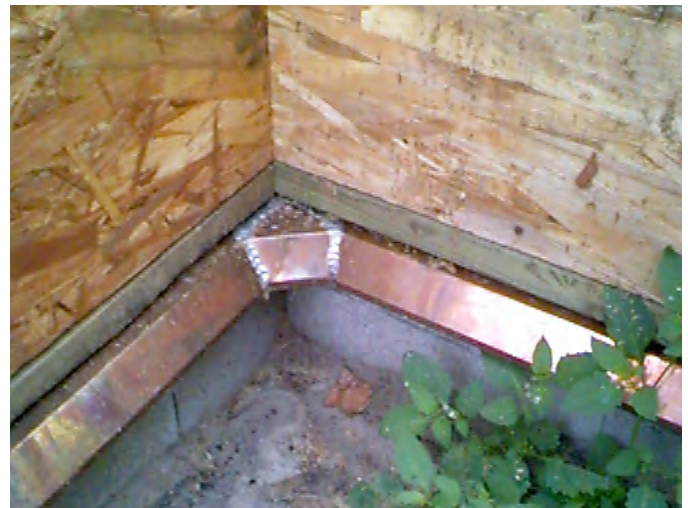
Figure 10 – Detail of metal shield at inside corner
