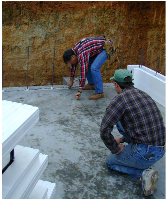
Figure 3 – Snap a chalk line to mark the wall layout
