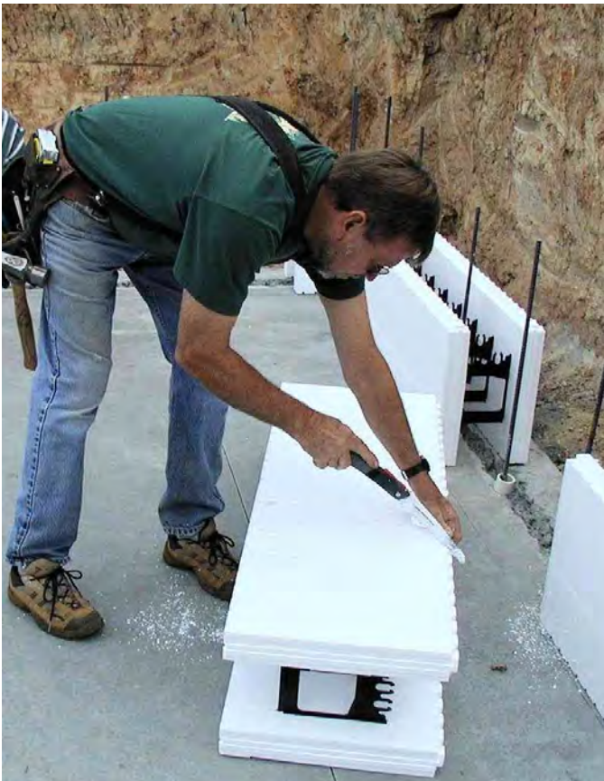
Figure 10 – Cutting the final block for a wall section
