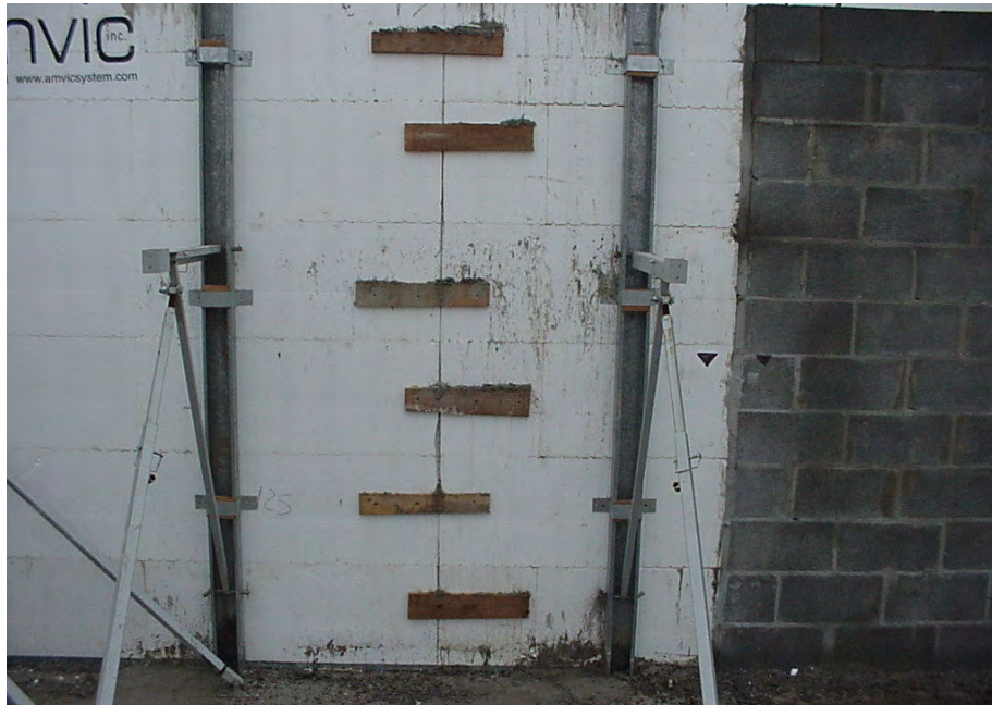
Figure 38 – Bracing a stack joint on both sides of wall
