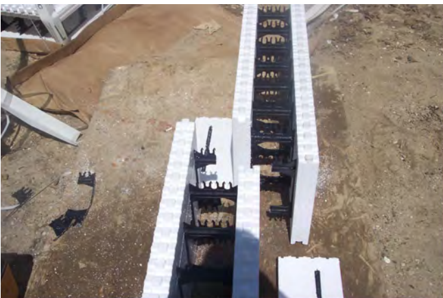
Figure 5 – Setting the two cut forms into position
