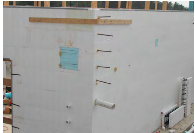
Figure 55 – Block opening voids with scrap foam or wood
