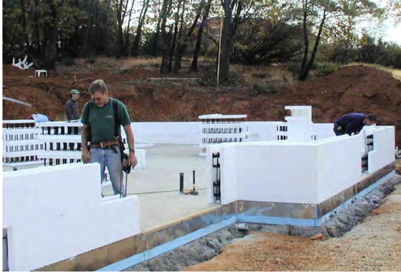
Figure 14 – Second course placement
