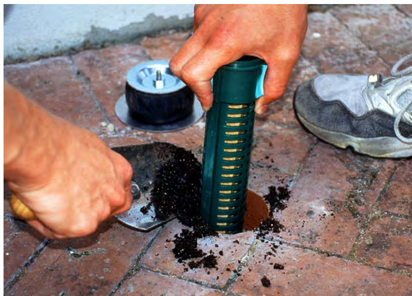
Figure 11 – Inserting a termite trap containing wood as bait
