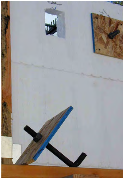
Figure 42 – Cutting square OSB boards for anchor bolt installation
