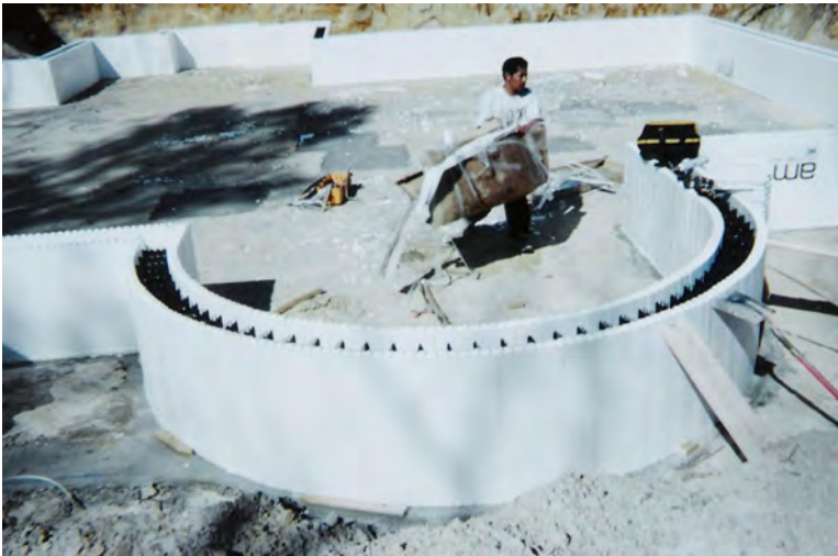
Figure 12 – Several courses of radius blocks installed
