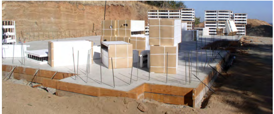
Figure 1 – Placing Amvic ICF within the perimeter of the wall layout
