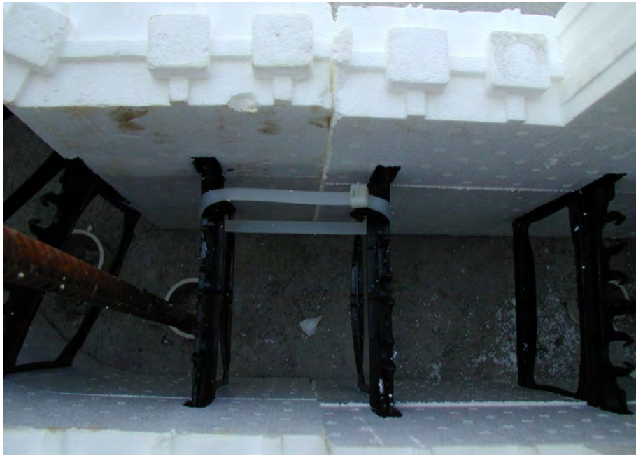
Figure 12 – Using zip ties to tie the first course of blocks together
