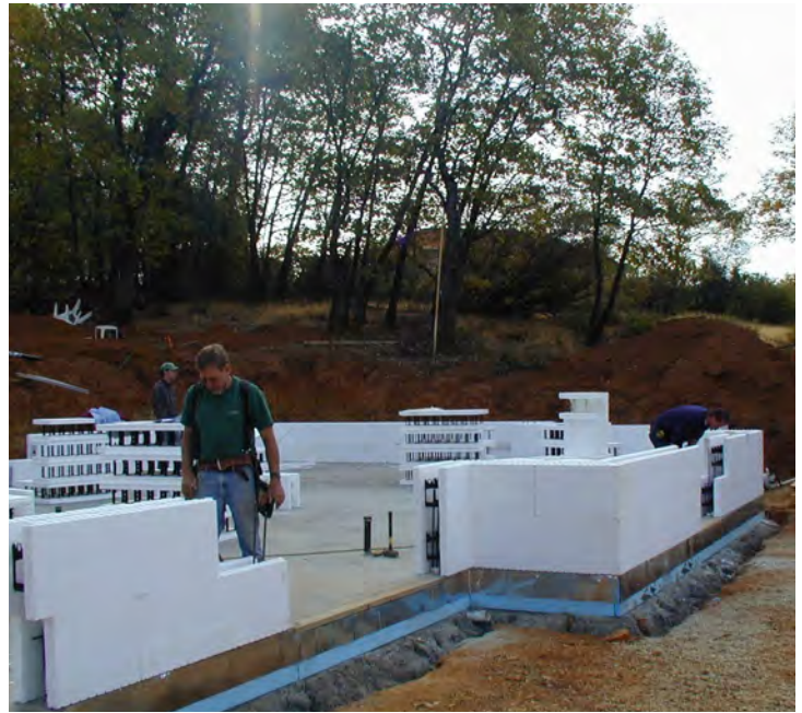
Figure 4 – Install second course of blocks
