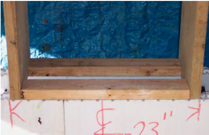
Figure 4 – Typical full width window buck bottom construction
