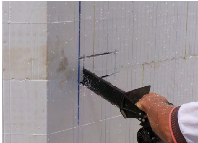
Figure 2 – Cutting a channel in the EPS panel using an electric chainsaw
