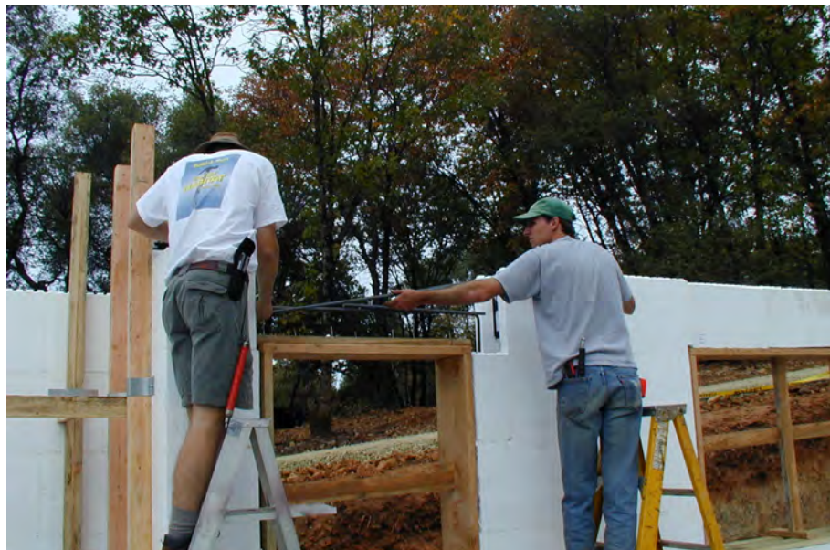
Figure 25 – Installing reinforcing steel bars for wall opening header or lintel
