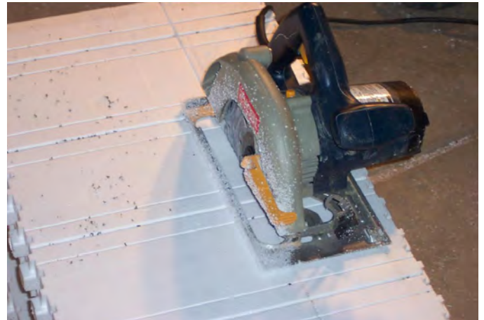
Figure 6 – Using a circular saw to horizontally rip cut ICF
