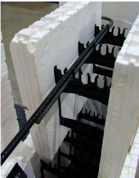
Figure 3 – Install horizontal reinforcing steel and lap splicing
