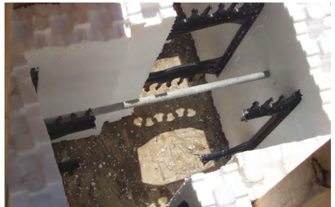
Figure 9 – Threaded rod inserted through both wood forms
