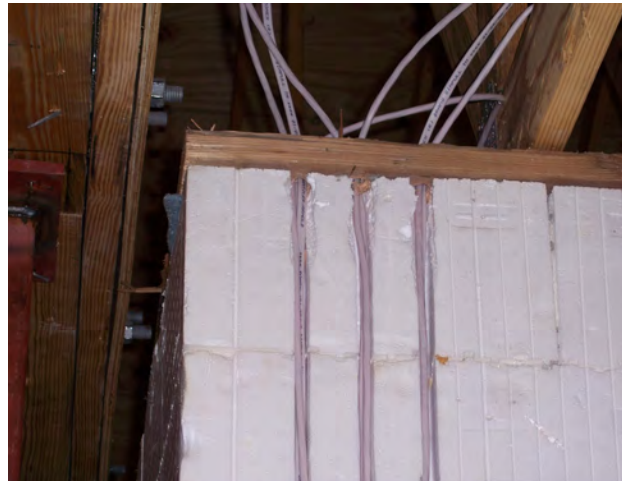
Figure 3 – Embedding Romex into the EPS panels
