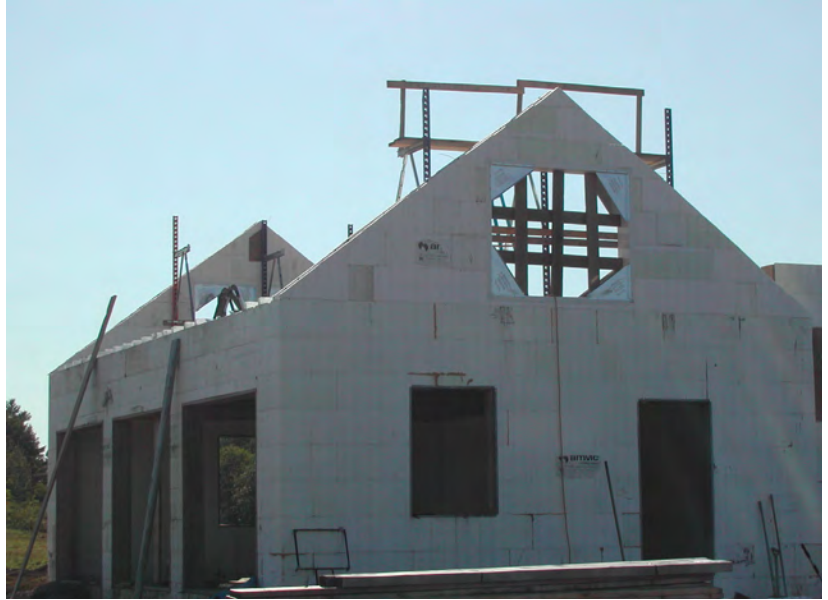
Figure 34 – Cutting forms to the shape of the gable end pitch
