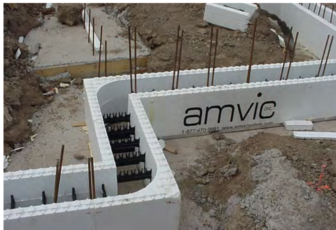
Figure 3 – Short corner made of 90° forms with a running bond pattern
