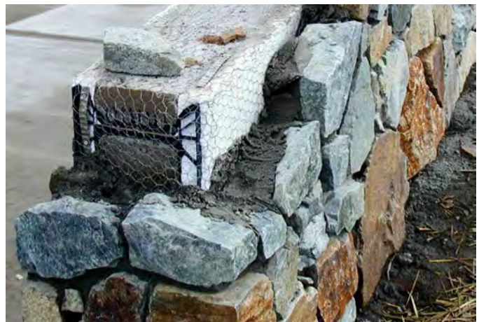
Figure 5 – Stone with ICF retaining wall
