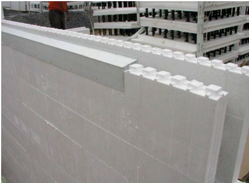
Figure 26 – Protecting the interlock on a top course
