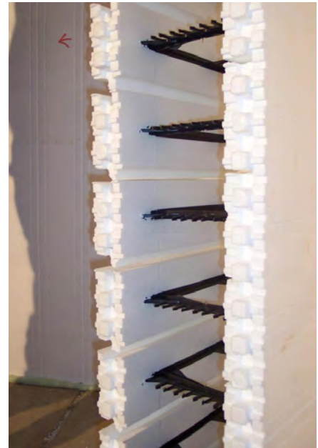
Figure 10 – Pre-cut Amvic radius blocks. Tongue and groove cut on the inside and slit cut on the outside
