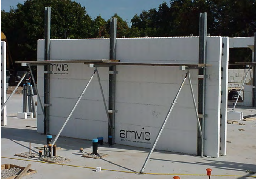
Figure 30 –Platform and scaffold planks
