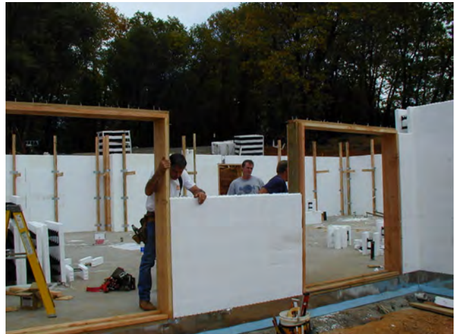
Figure 22 - Stacking courses around door bucks
