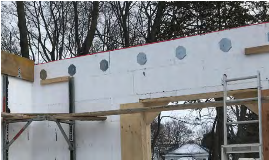
Figure 51 – Securing the ledger board in place temporarily
