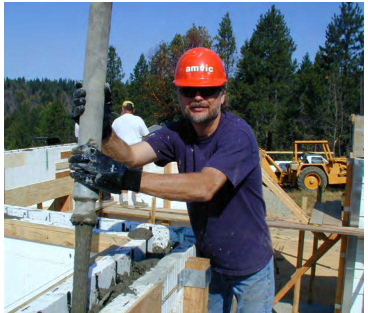
Figure 9 – Pour concrete in lifts of 3-4' (0.9-1.2m)
