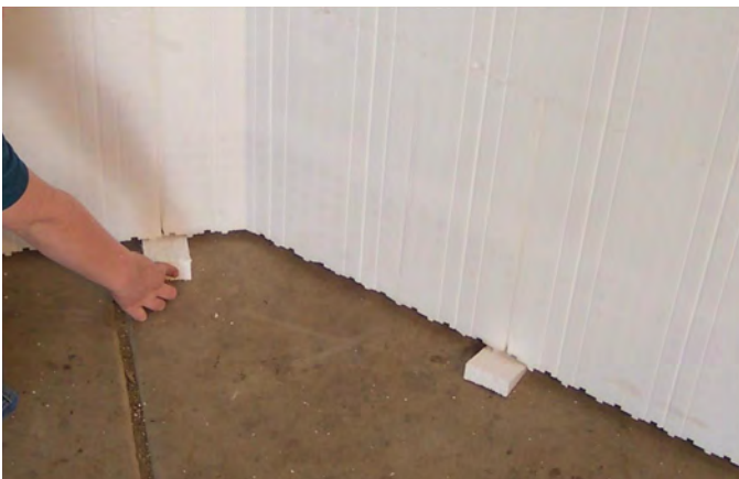
Figure 18 – Shimming the first course with foam cuttings
