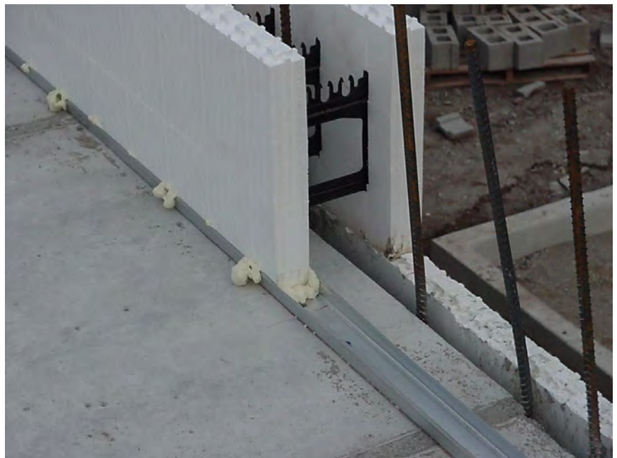
Figure 5 – Metal track section acting as a guide for block placement
