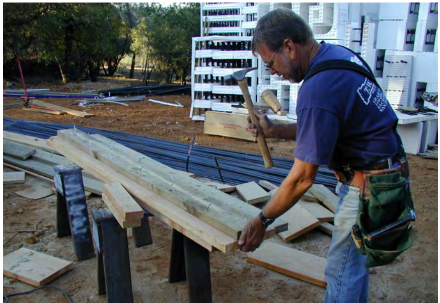
Figure 6 – Installing nails into the buck for attachment to concrete
