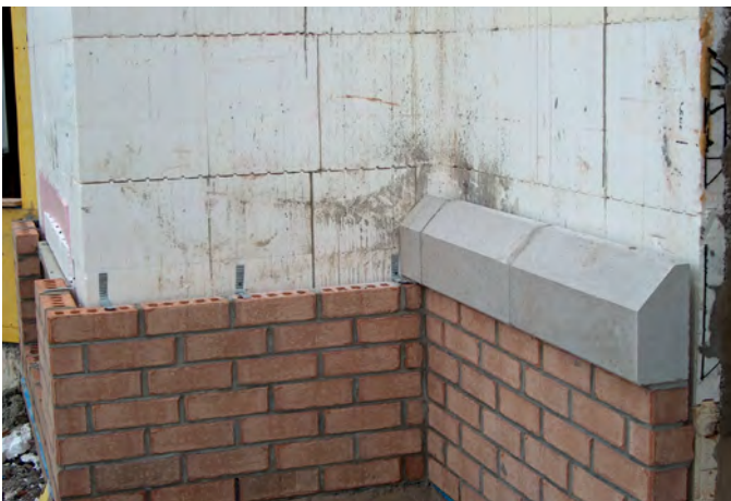
Figure 4 – Brick veneer construction with Amvic ICF
