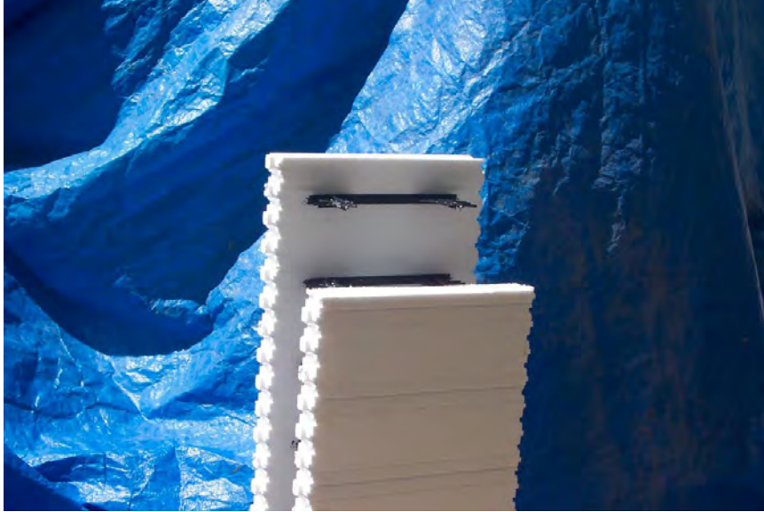
Figure 4 – Cutting foam from the end of the straight block on one EPS panel
