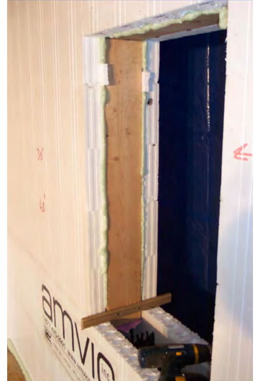
Figure 35 – Filling gaps between bucks and forms with foam adhesive
