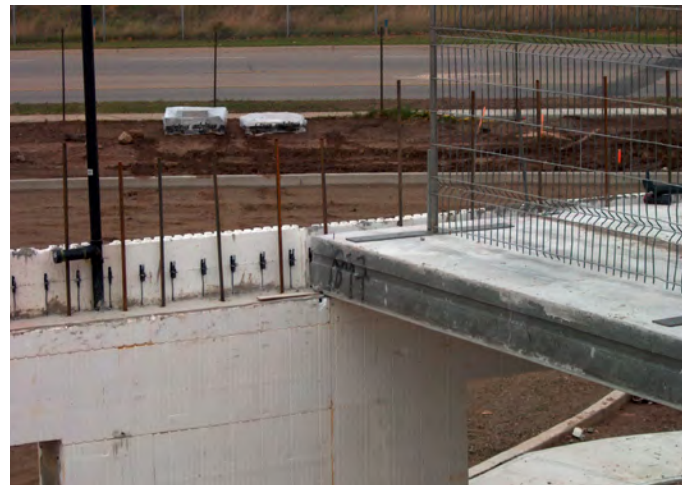
Figure 36 – A precast slab panel placed on an ICF wall
