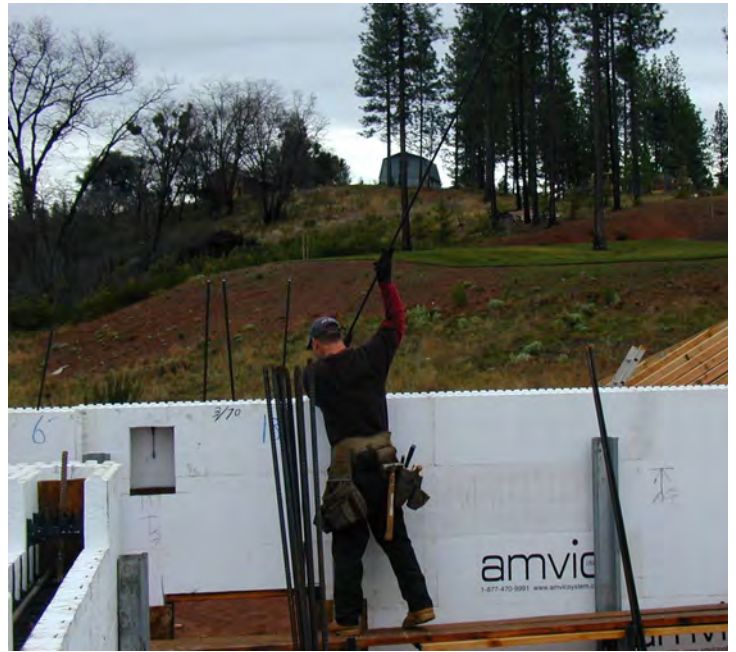
Figure 8 – Install vertical reinforcing bars after top course of blocks
