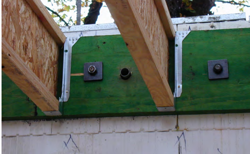
Figure 47 – Installing ledger board with proper nuts and washers
