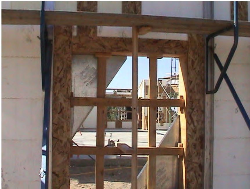
Figure 37 – Bracing wall opening vertically and horizontally
