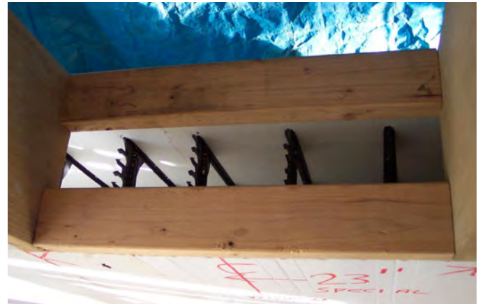
Figure 5 – Opening at bottom of full width window buck for pouring concrete
