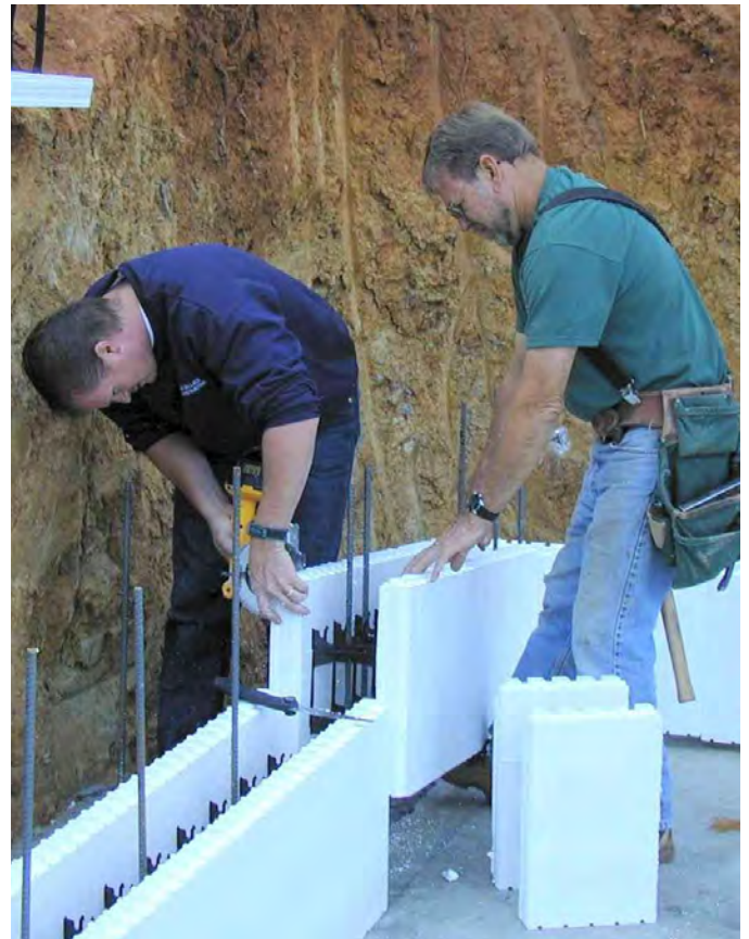
Figure 11 – Fitting the cut block in place
