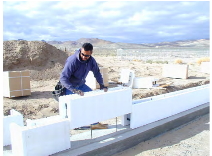
Figure 9 – Placing straight blocks
