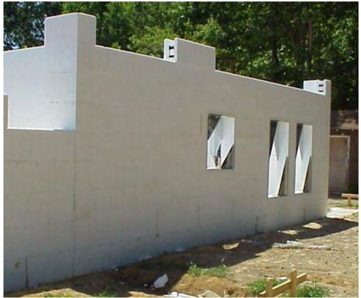
Figure 6 – Continue installing block courses
