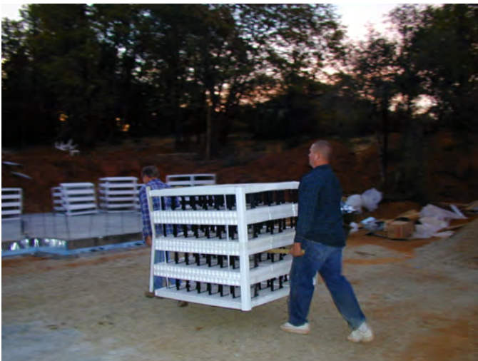
Figure 2 – Moving ICF bundles by hand
