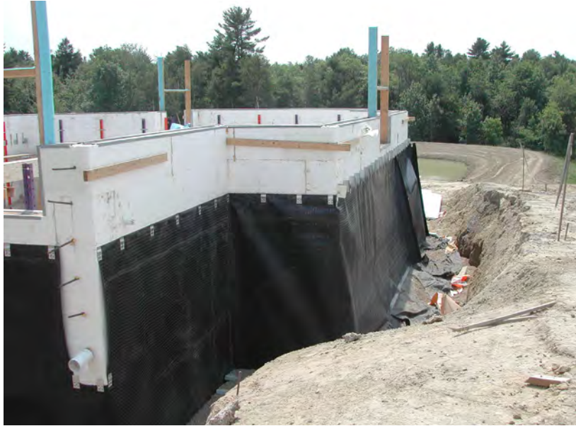
Figure 5 – Installed dimpled membrane on Amvic ICF foundation
