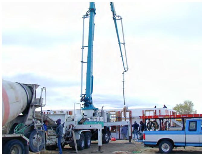
Figure 7 – Using boom pump to pour concrete in Amvic ICF
