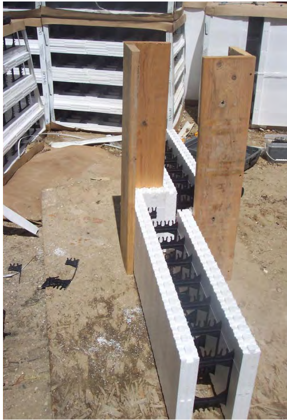
Figure 7 – Using 2x10" (38x235mm) wood forms to support the formed corner
