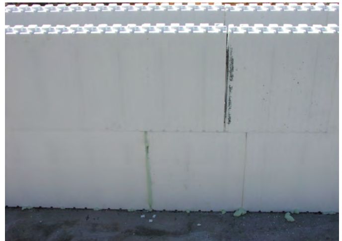
Figure 16 – Placing the offset joint in approximately same place as first course
