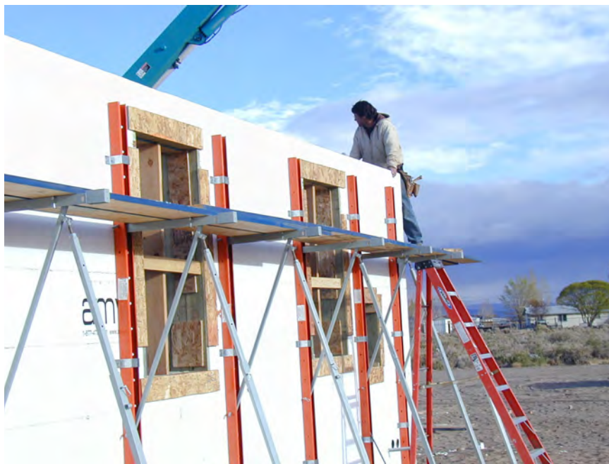
Figure 33 – Bracing both sides of wall openings
