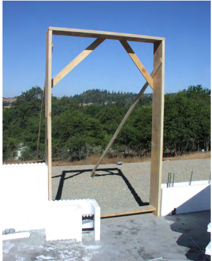
Figure 7 – Placing Door Bucks
