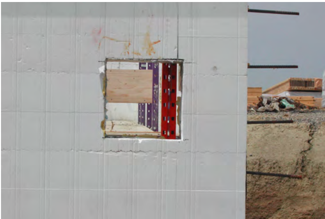
Figure 54 – Cut beam opening through both EPS panels
