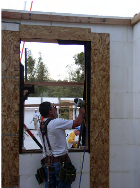
Figure 40 - Cleat installation around a door opening using OSB
