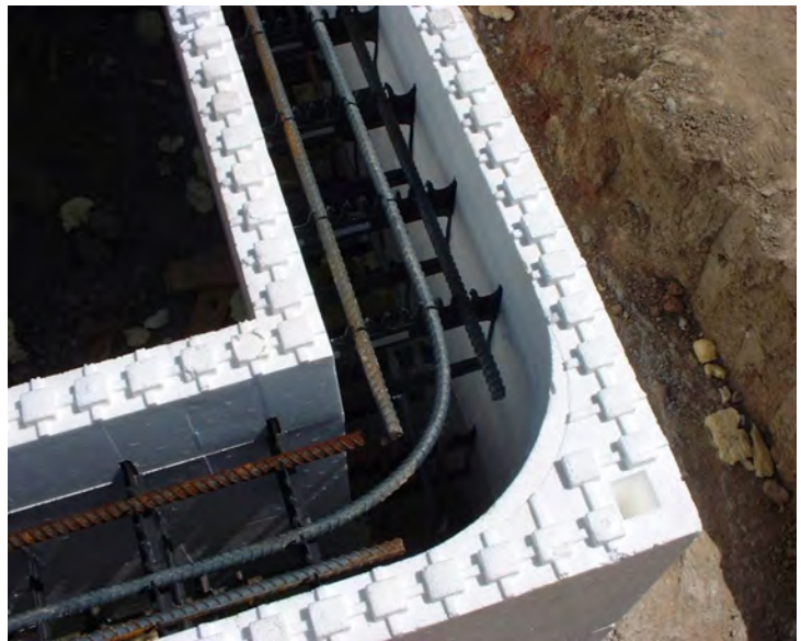
Figure 2 – Place corner blocks first
