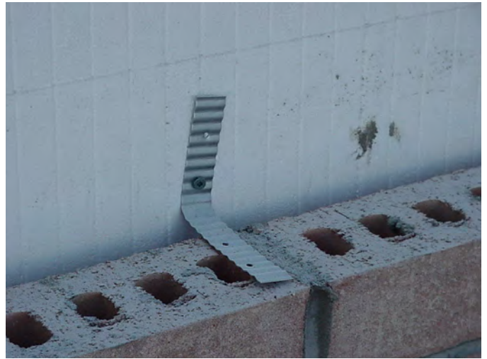
Figure 25 – Standard brick ties screwed into the Amvic webs
