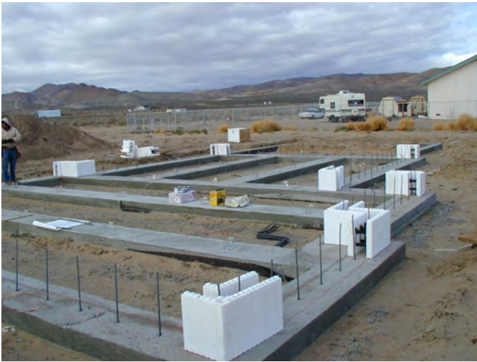
Figure 8 – Placing corner block first
