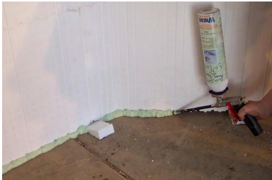
Figure 21 – Gluing an unshaven first course to the footing/slab
