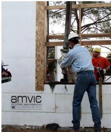
Figure 9 – Pouring concrete at window sills
