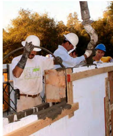
Figure 10 – Using internal vibrator to consolidate concrete
