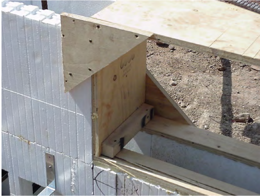
Figure 36 – Installing cleats around wall openings
