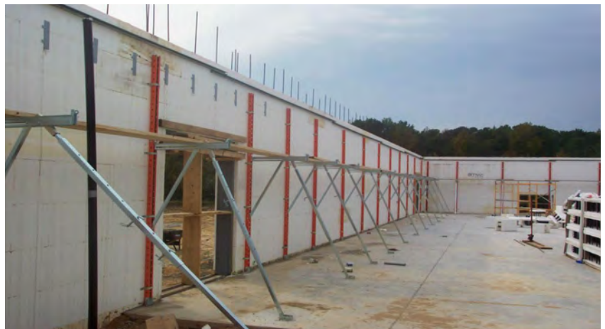
Figure 29 – Bracing on the inside of the wall
