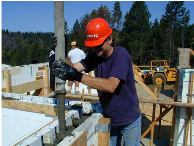
Figure 8 – Pouring concrete for 90° corner
