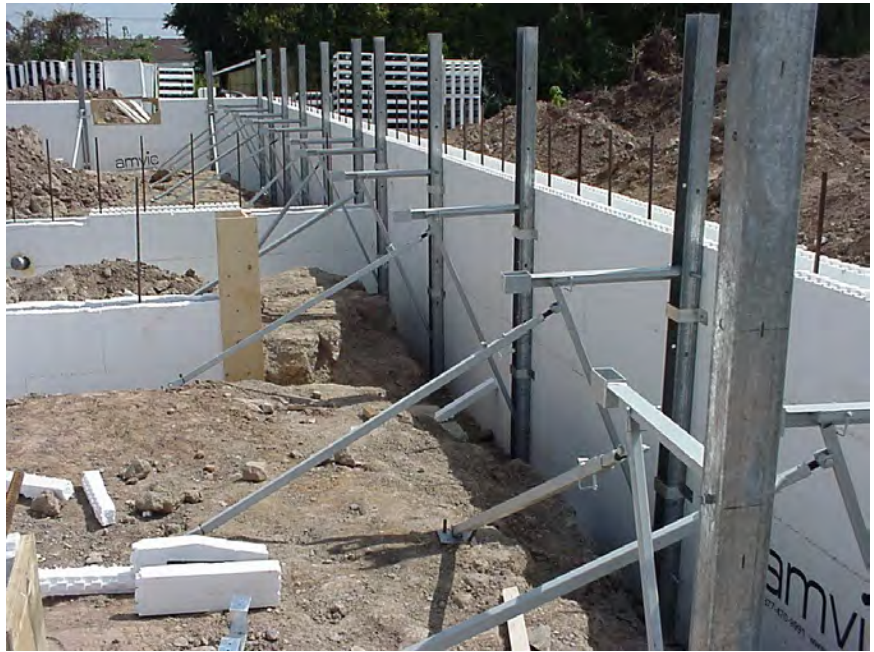
Figure 34 – Bracing every 6' (1.8m)
