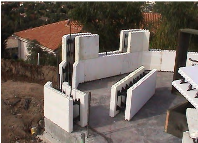
Figure 15 – Reversing 45° corner blocks for bay window
