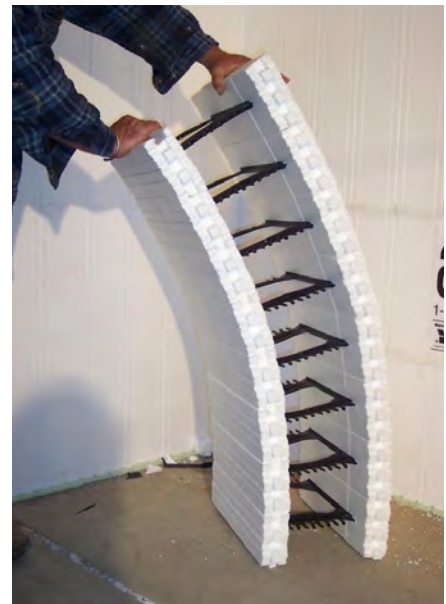
Figure 11 – Bending and securing the radius form into place
