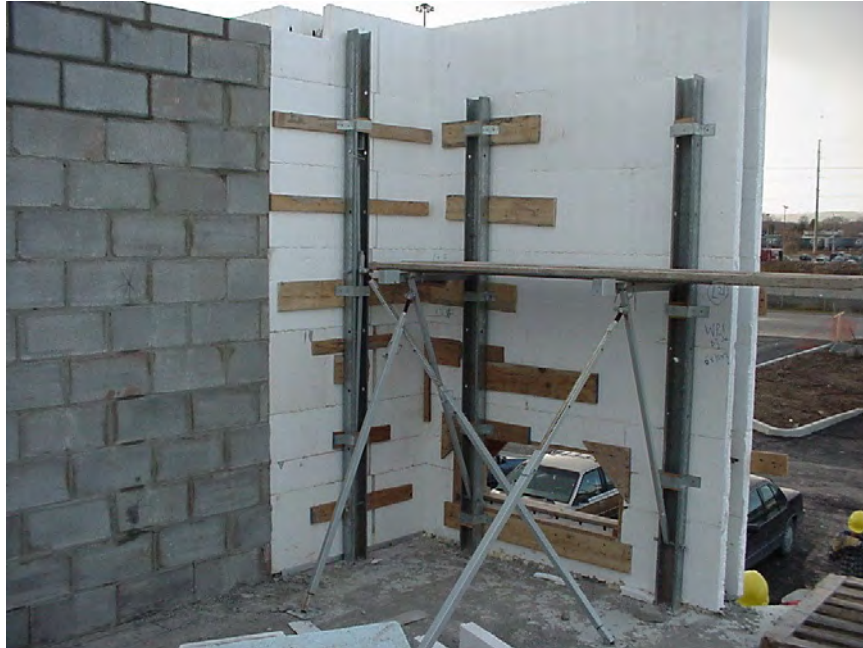
Figure 32 – Bracing corners on the inside
