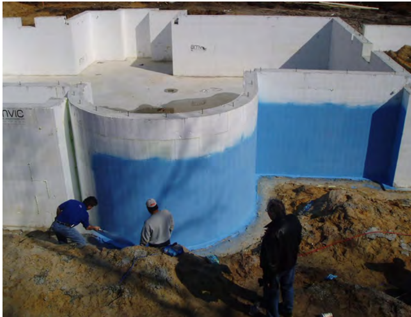
Figure 3 – Spraying liquid applied membrane on Amvic ICF
