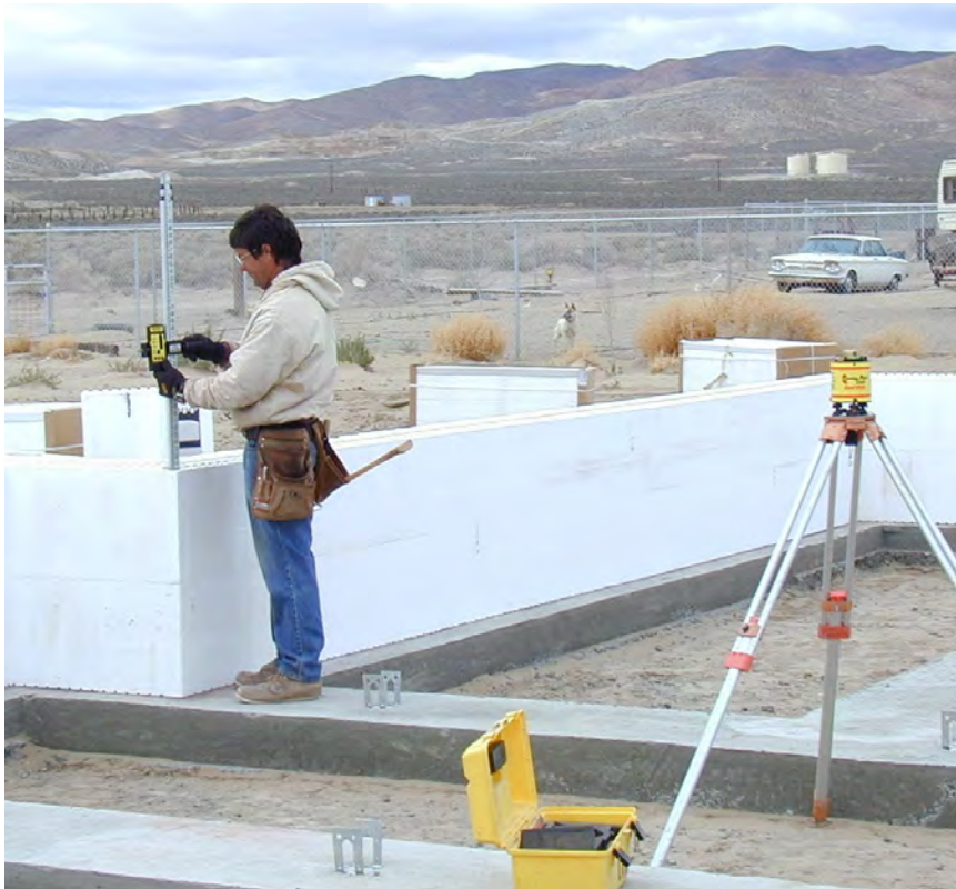
Figure 17 – Checking for level after second course placement
