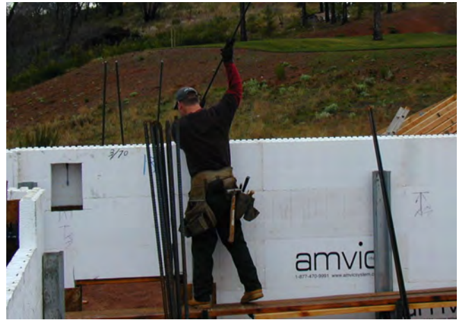
Figure 27 – Installing vertical rebar
