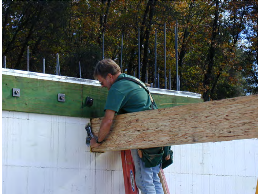
Figure 58 – Maneuvering wood beam in place to bear on beam pocket
