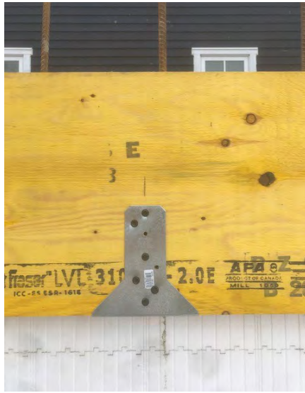
Figure 52 – Laminated Veneer Lumber ledger attached using ICFVL-CW
