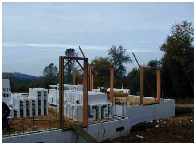
Figure 23 - Installing Door bucks on the second floor
