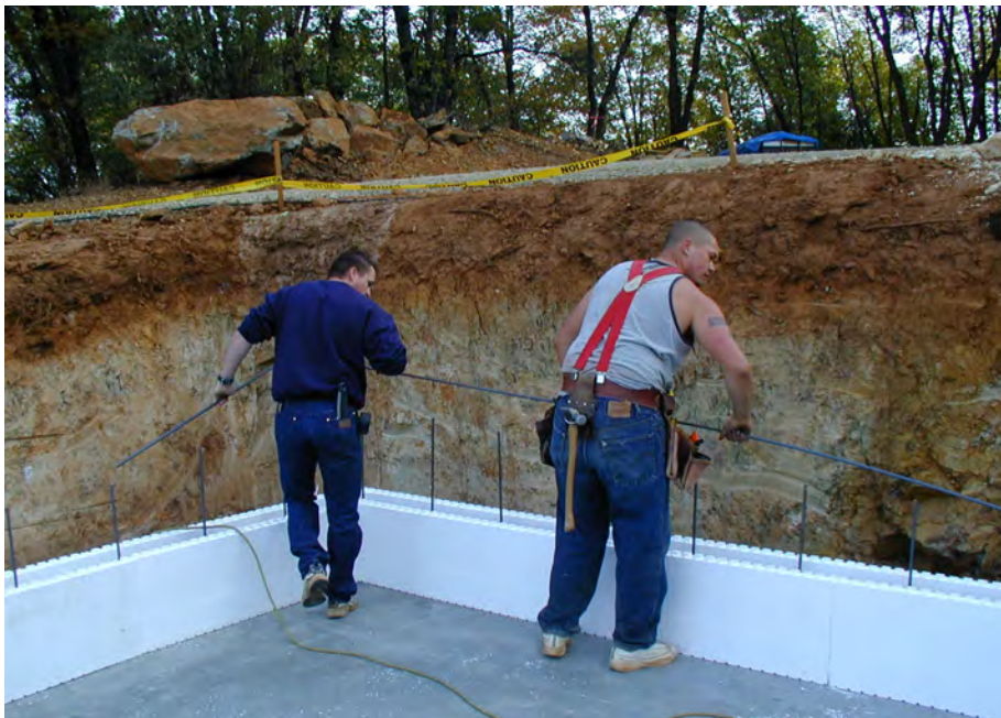
Figure 13 – Installing horizontal rebar
