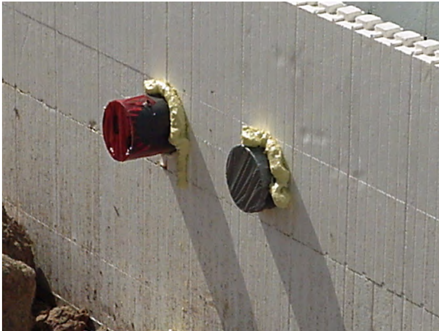
Figure 41 – Using PVC pipe for penetration block-outs
