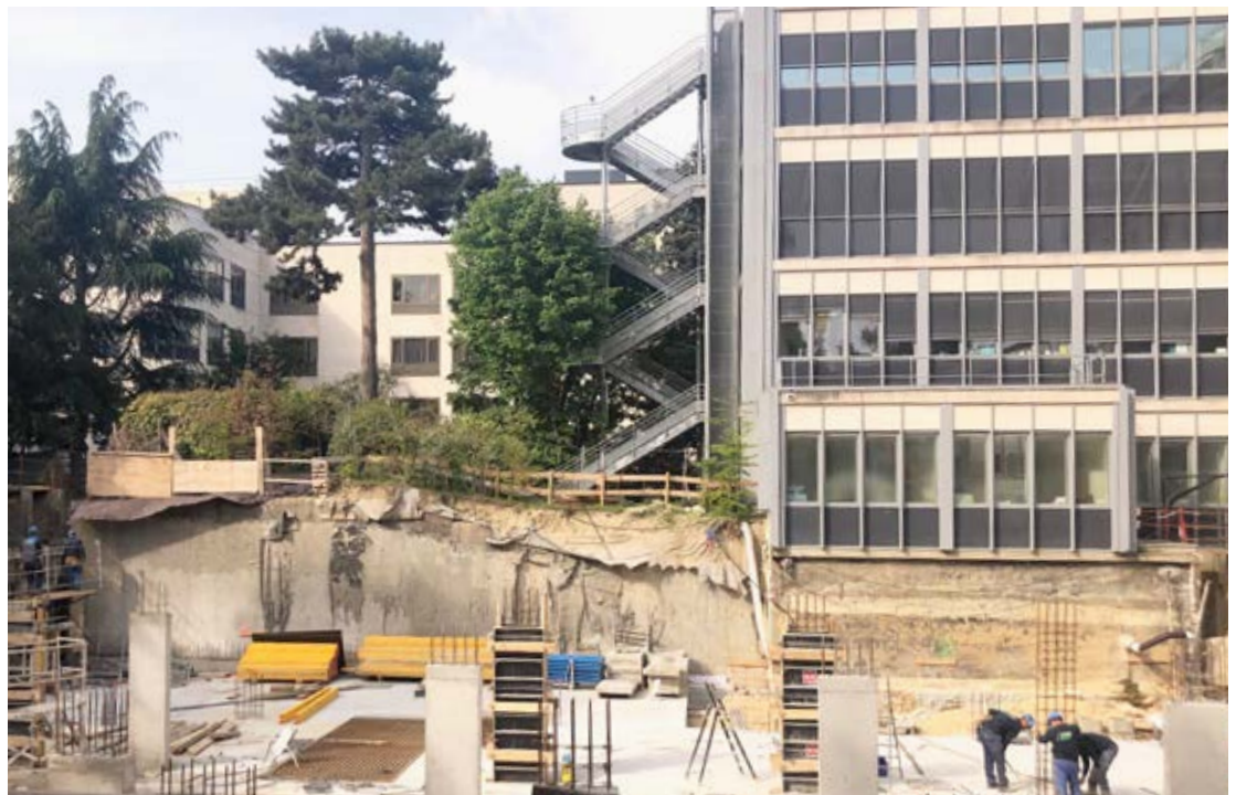
The construction site of our Medical Imaging Center
