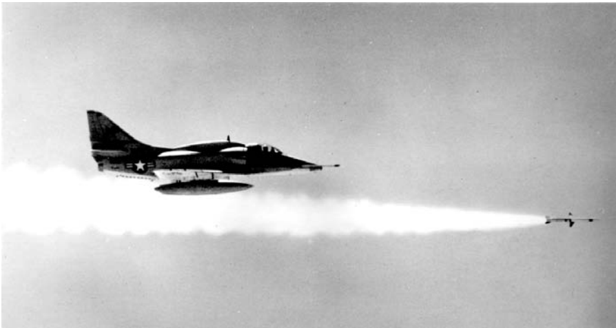
Figure 60. Navy A-4 firing Shrike. An active counter to Communist radar was the Navy's Shrike antiradiation missile that homed in on radar signals. It was also used by the US Air Force. (Reprinted from USAF.)
