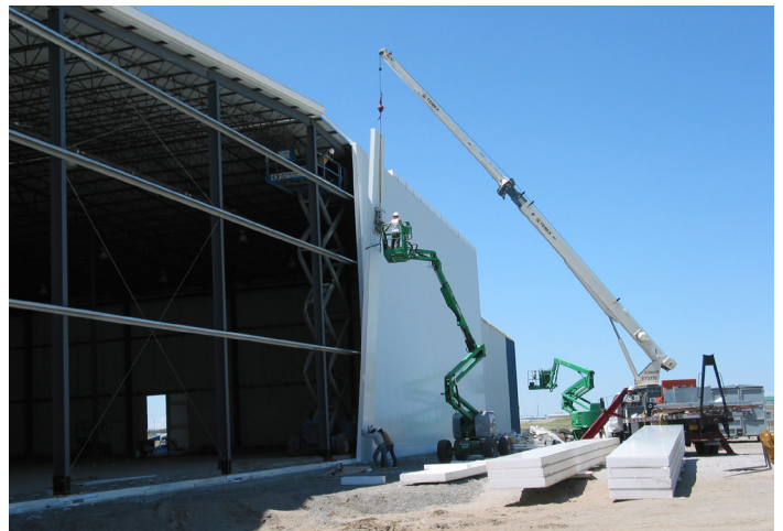
Installation of a vegetable freezer in Washington state
