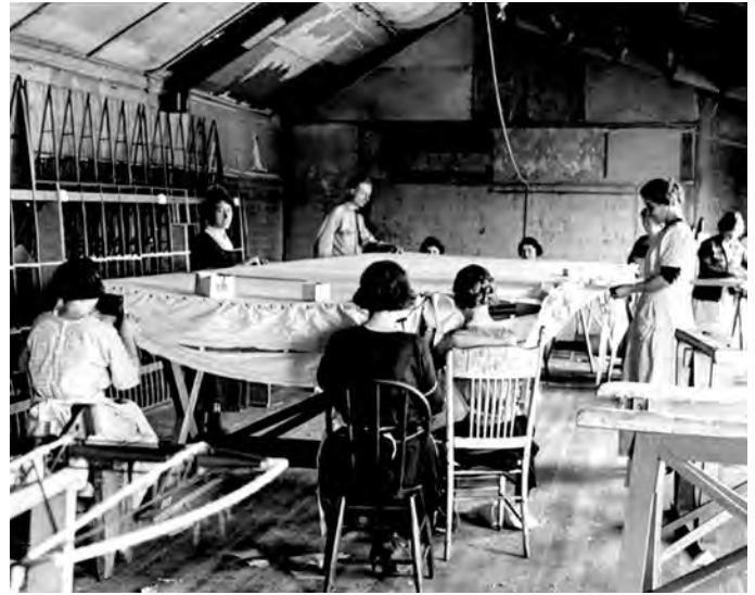
Placing canvass on the Douglas aircrafts' wooden frame.
