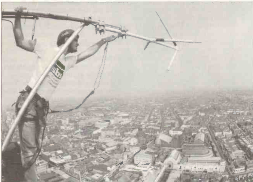
sbs project engineer Dave Stanley goes out on a limb.
