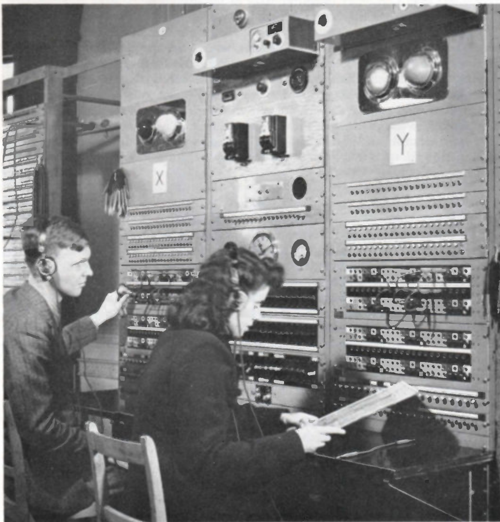
Programme distribution switching at the External Services centre at Aldenham, Hertfordshire (1943 to 1952)
