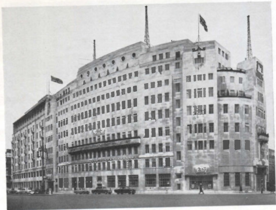
Broadcasting House, London, showing the Extension on the left in which new technical and programme facilities have been provided. These were brought into use progressively during 1961
