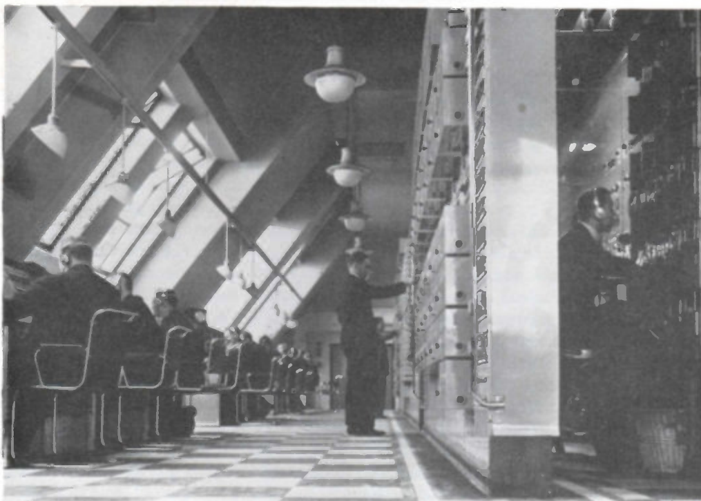
Broadcasting House, London Control Room showing amplifier racks and transmission position (1932)
