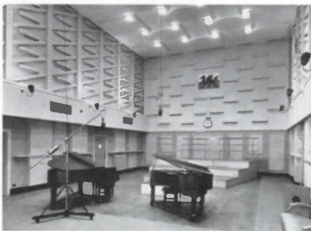
Studio 1, Swansea, showing cavity absorbers
