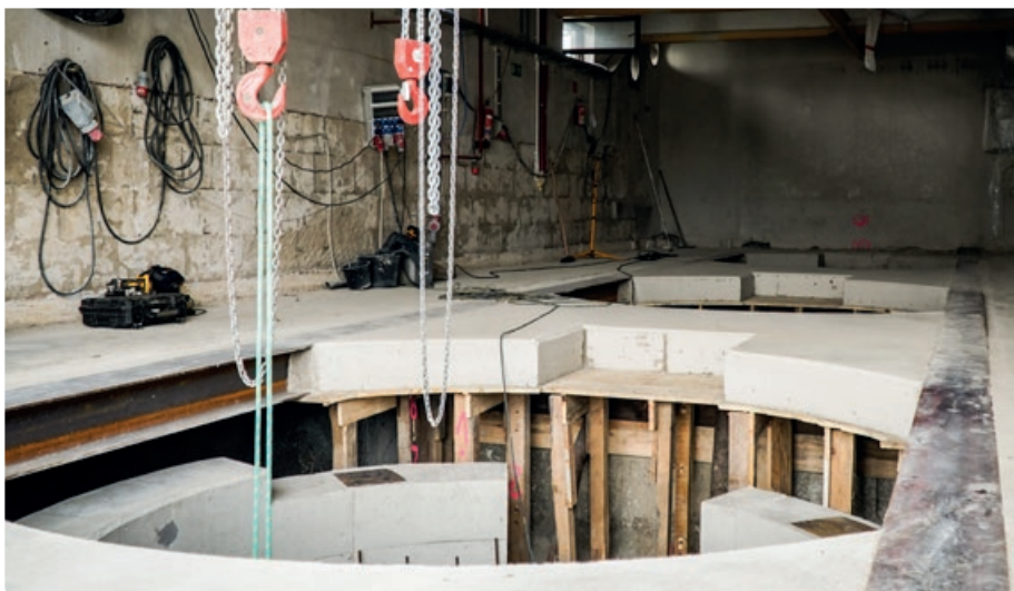
Fig. 5. From top: turbine cases awaiting installation, turbine chambers
