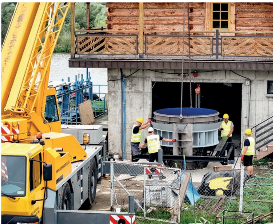
Fig. 3. Installation of the Kaplan turbine case
