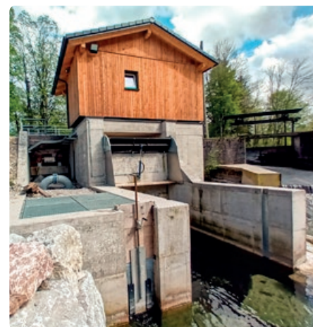
Fig. 4. Fishcon lock Schwarzmühl at the river Alm next to the residual flow power plant
