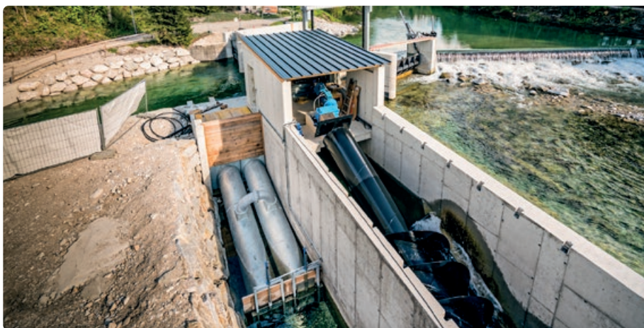
Fig. 3. Fishcon lock Lippenannerl at the river Alm next to the residual flow hydroelectric screw turbine
