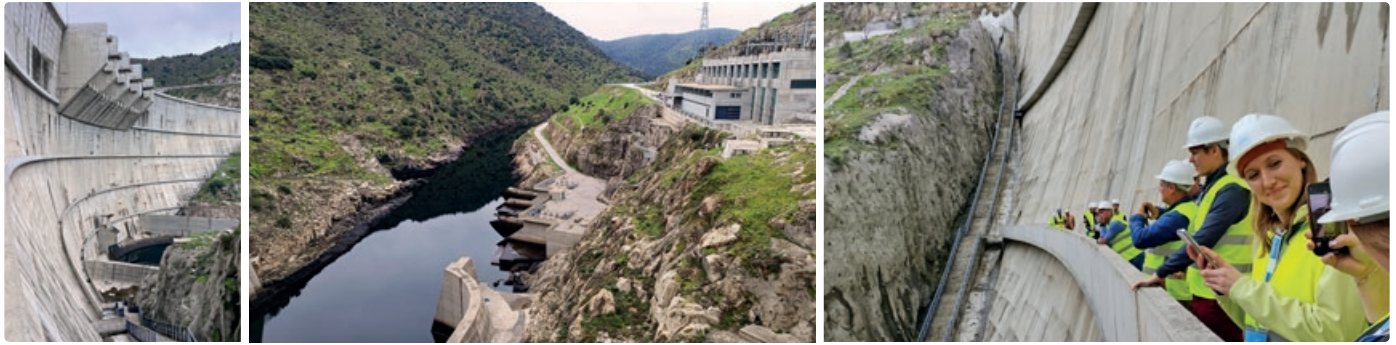
Fig. 2. PSH Baixo Sabor, from left: view of the dam from the downstream side with the spillway, power plant building with discharge channels, participants of the study tour visiting the dam from the technical terrace level
