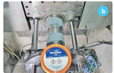
Photo 2. Refurbishment using BELZONA(1111) composite: a) shaft journal, b) roller bearing housing
