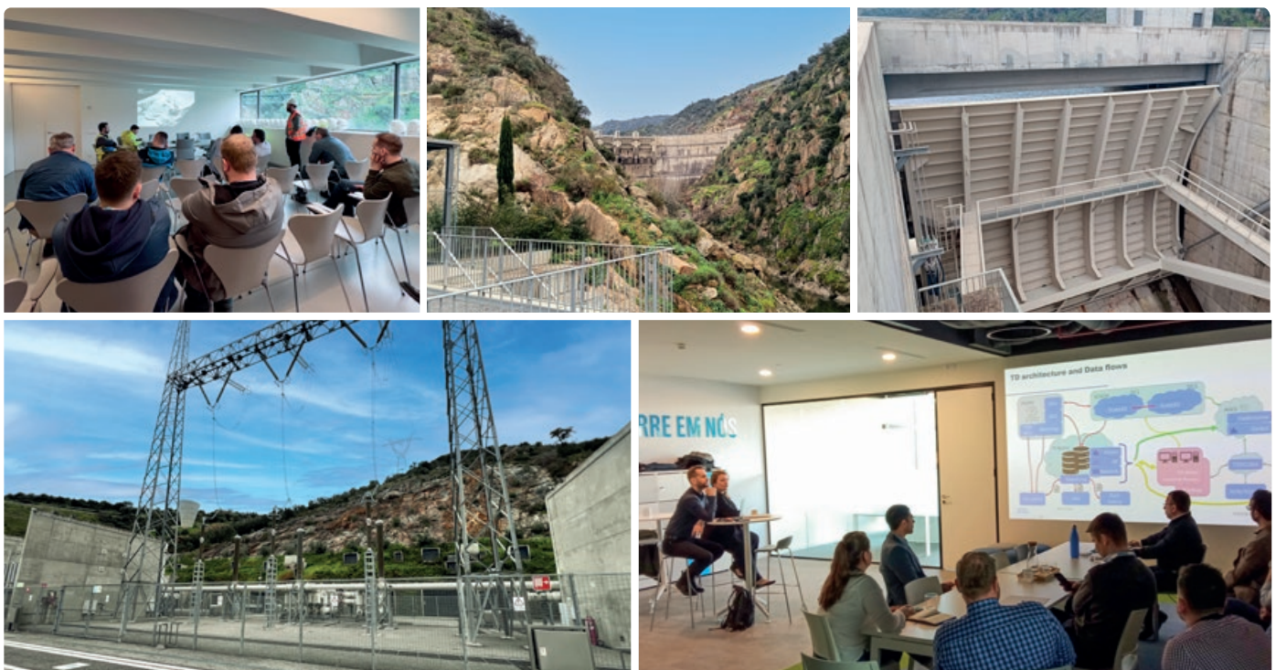
Fig. 3. PSH Foz Tua, from left: briefing of study tour participants before visiting the facility, the Tua river valley with the dam, segment gate of the spillway, transformer station, workshops at Engie headquarters – presentation on the management system of hydropower plants
