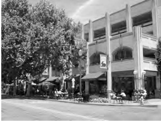
Figure 4.2.18: This parking structure is accessed from a side drive allowing commercial establishments to front the street and activate the sidewalk.
