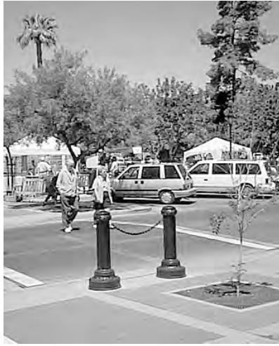
Figure 2.2.3: Bulb-outs and diagonal parking narrow the width of street crossings giving pedestrians a sense of belonging even while crossing the roadway.
