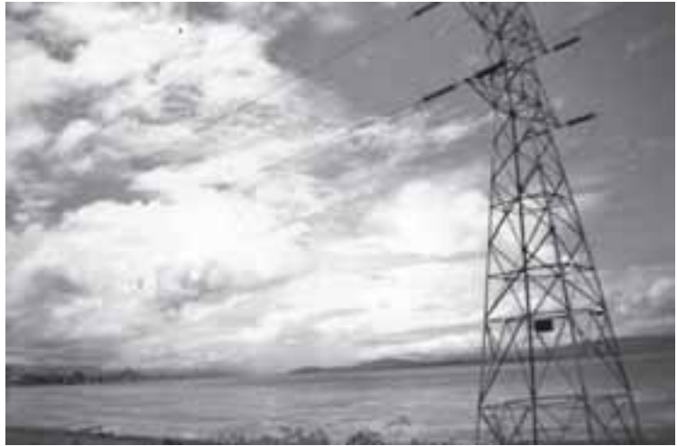
A power pylon overlooks Moby reservoir Photo: KDRG
