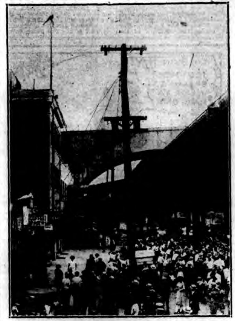
"Daredevil" on Kindred Building Flagpole; Connecting Railroad Viaduct in Background.
