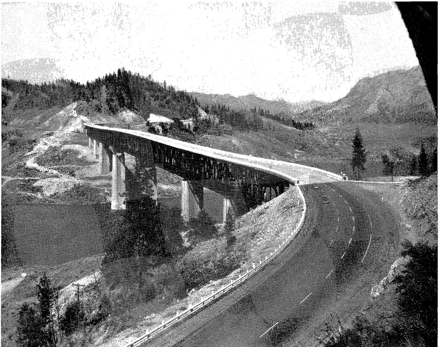
Pit River Bridge across Shasta Lake (still being impounded at time this picture was taken). This is one of the few structures which carries both highway and railroad traffic.
