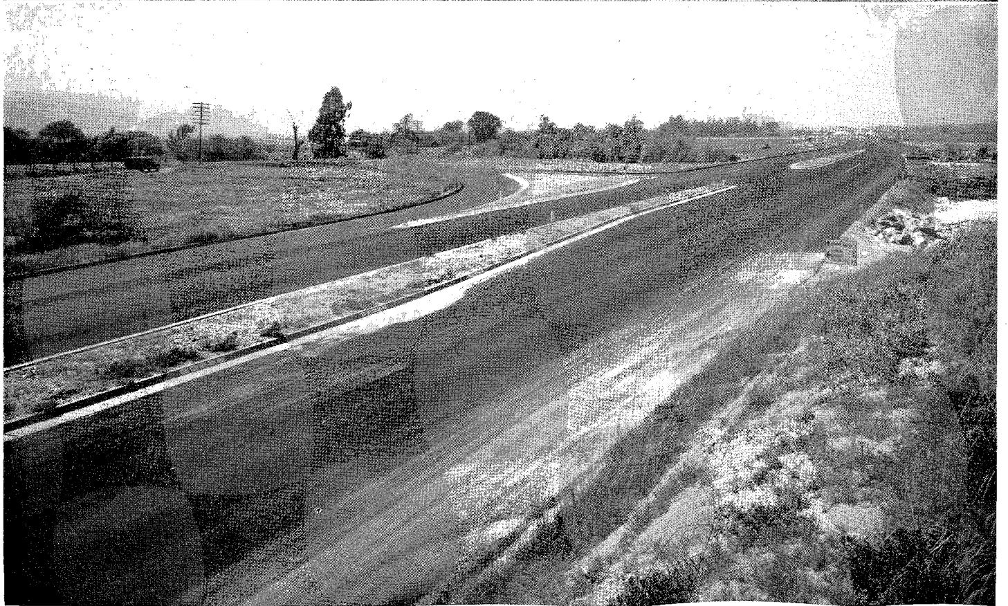
Upper—One of two 90 degree turns on U. S. 395 and Adelanto, typical of deficiencies in the Mojave Desert portion of U. S. 395. Lower—Junction of old and new U. S. 395 one mile north of Temecula, looking northerly along the Temecula-Antelope road unit recently completed.
