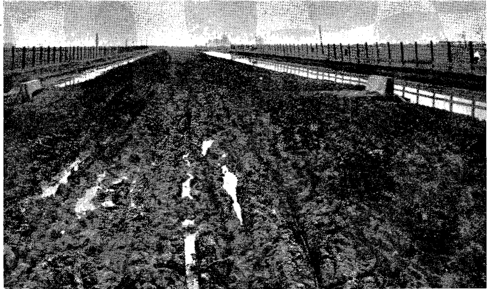
This road in Sacramento County was typical of many which confronted the first California Highway Commission in 1911.
