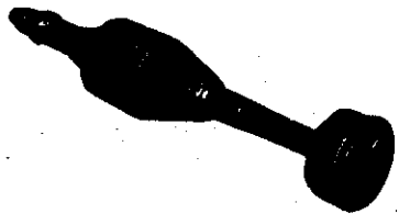
Figure 1.—8.8-cm antitank hollow-charge projectile (4312).
