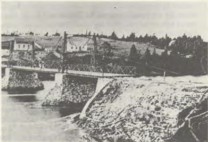
Bridge construction at Colinet
