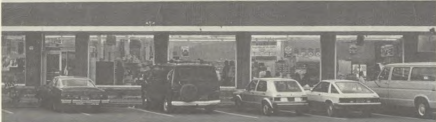
Gander Co-op building
