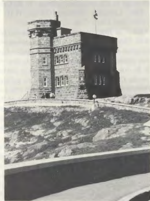
Cabot Tower on Signal Hill
