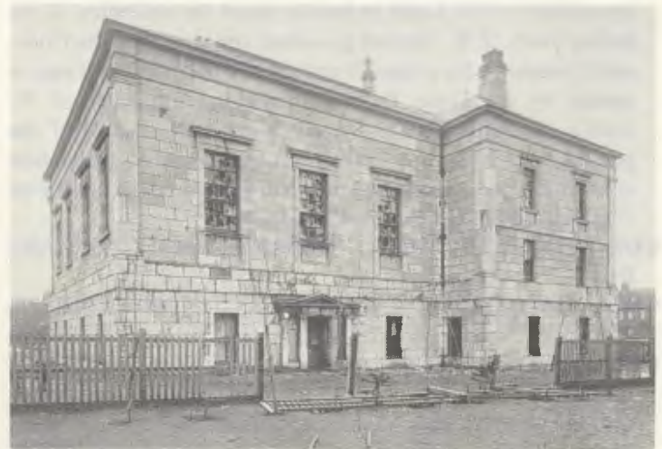
Colonial Building after 1932 riot.
