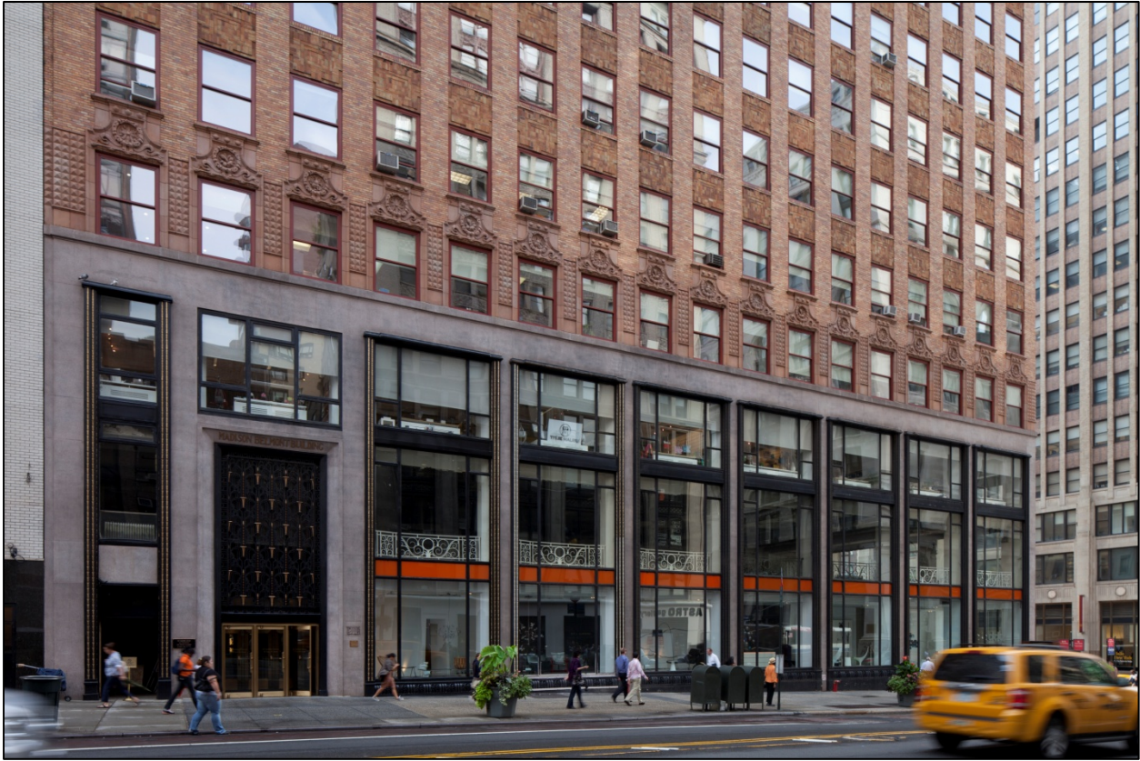
Madison Belmont Building 34 th Street, lower floors Photo: Christopher D. Brazee, 2011
