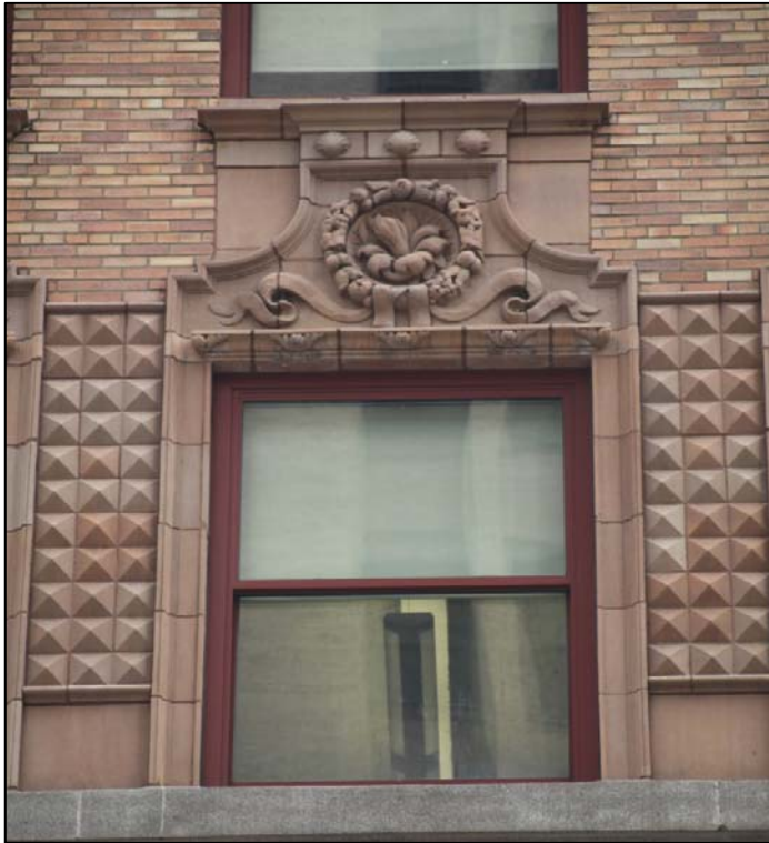
Madison Belmont Building Brick and Terra Cotta details Photos: Christopher D. Brazee, 2010
