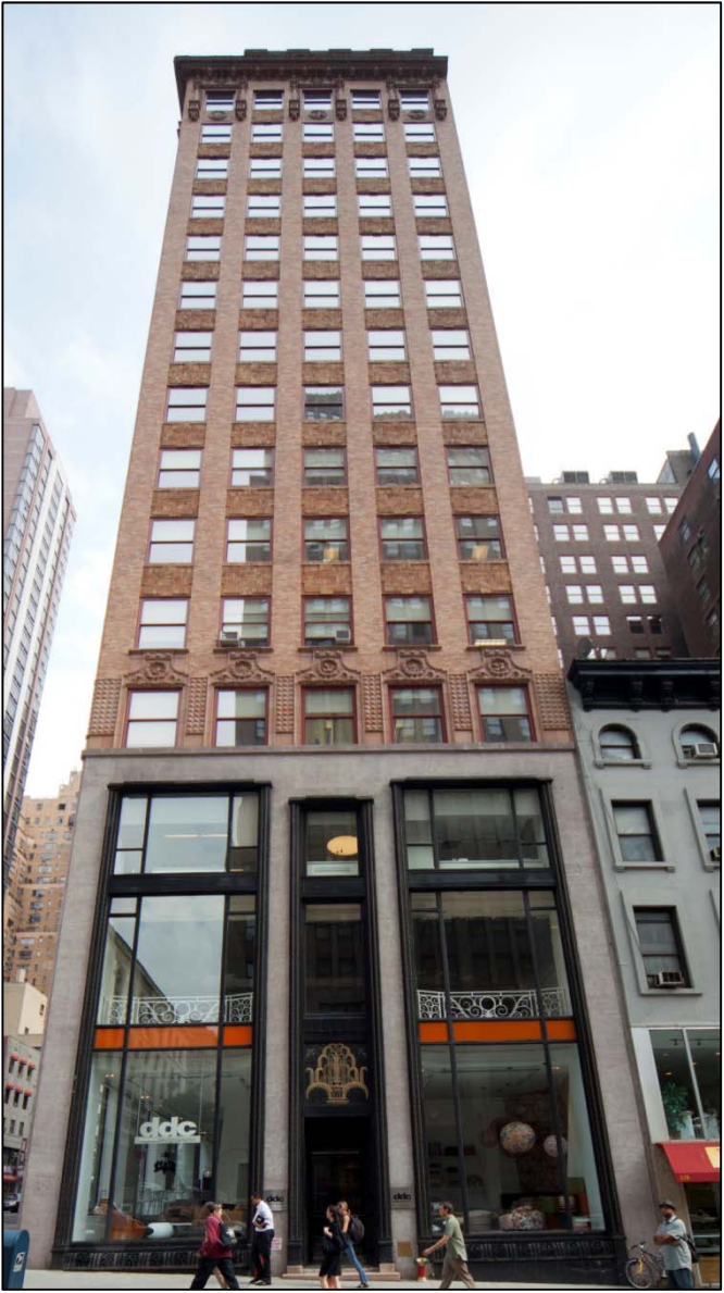
Madison Avenue facade
