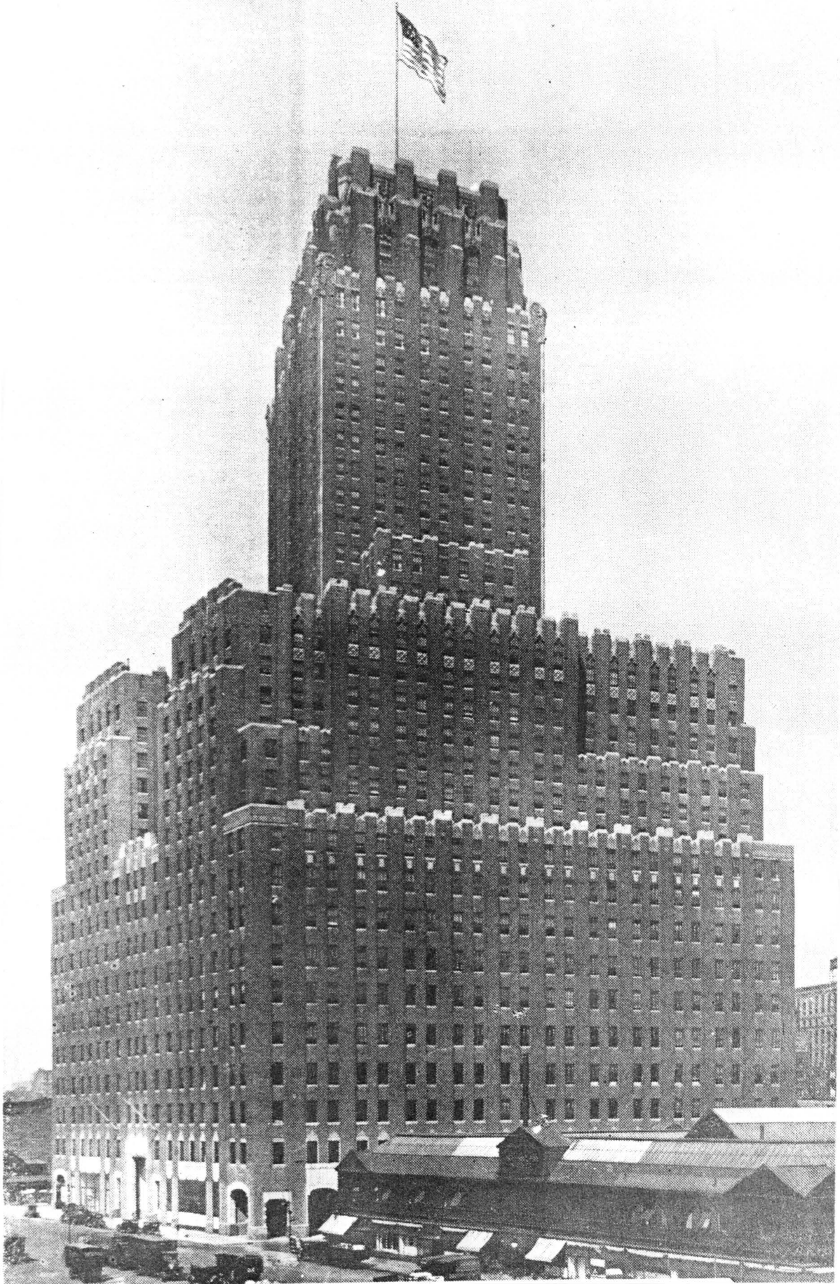
Fig. 10: Historic view of the Barclay-Vesey Building from the south showing the Washington Market in foreground. (New York Historical Society, Postcard Collection.)
