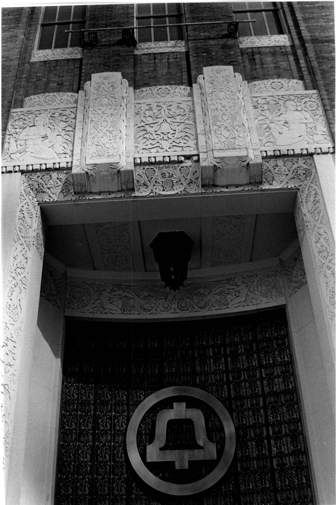
Fig. 9: Entrance detail. Note light fixture and limestone detailing. (Photo Credit: Carl Forster.)
