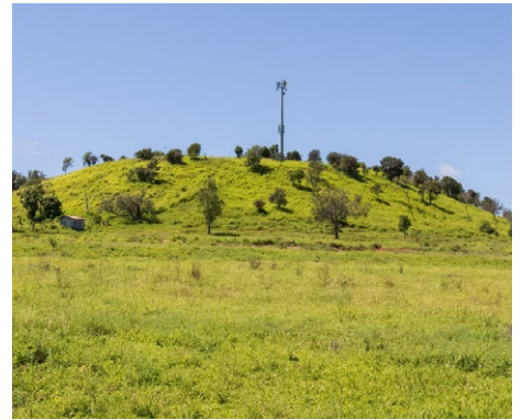
Transmission towers on the hill south of the town
