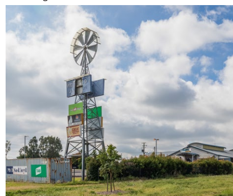
Westbrook Junction windmill is a key landmark and highly evident when viewed from Toowoomba-Athol Road (A139)
