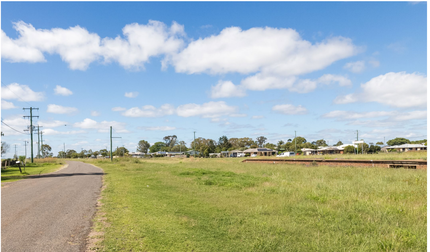
View along Hartvigsen Street showing the former Wyreema Station platform
