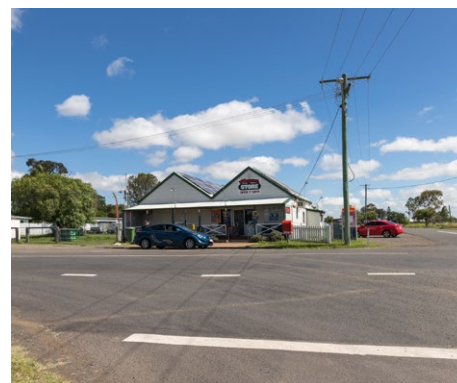
Informal parking adjacent to the general store
