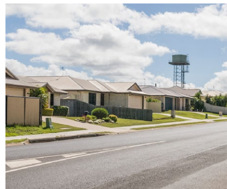
The water tower on Cashmore Street acts as a local landmark
