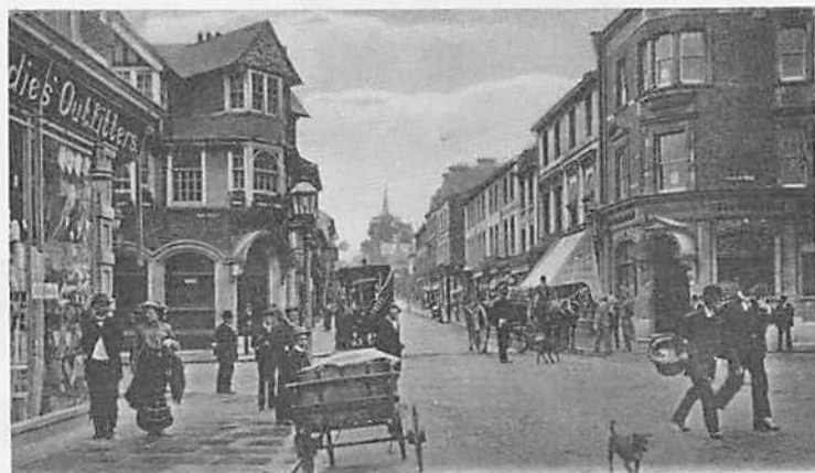
Fig. 5. Redhill, Station Road.
